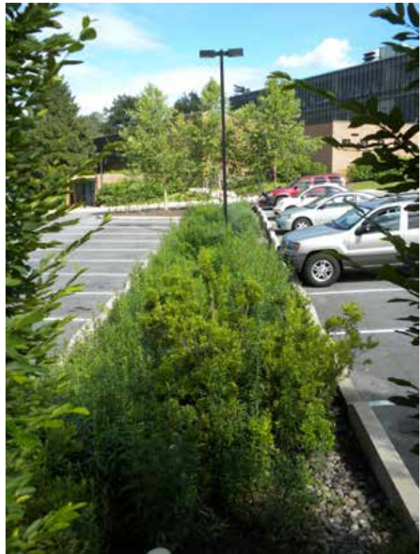
Example of stormwater management integrated into a parking lot.
