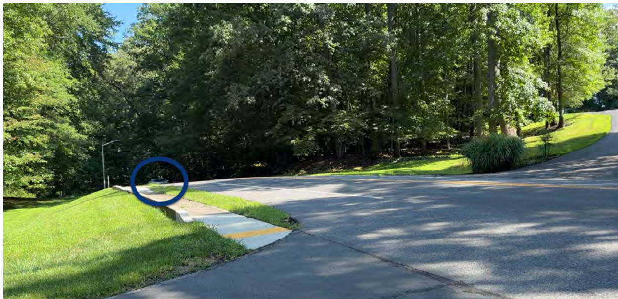
Figure 3. Observed Sight Distance – Valentine Creek Drive at Old Herald Harbor Road
