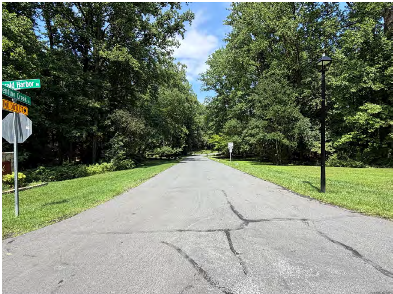
Figure 2. Valentine Creek Drive at Old Herald Harbor Road (Northbound)
