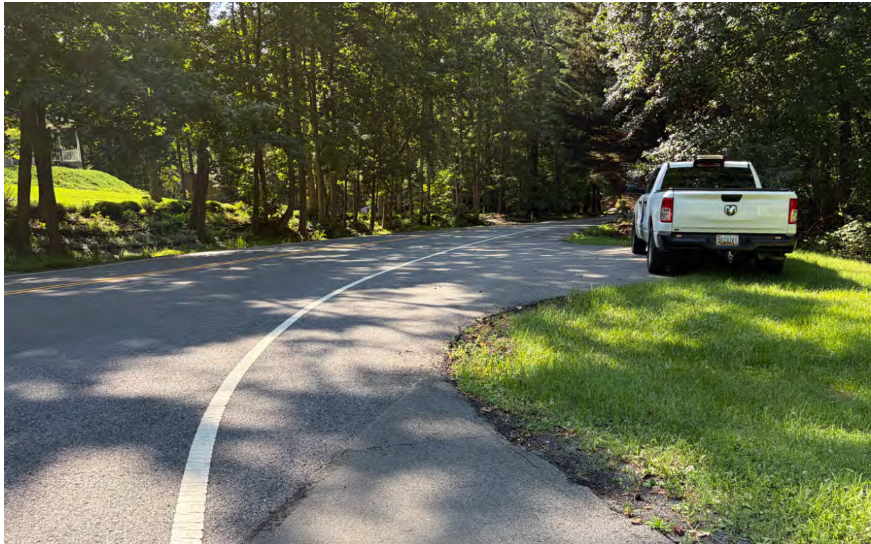
Figure 4. Observed Sight Distance – Valentine Creek Drive at Old Herald Harbor Road
