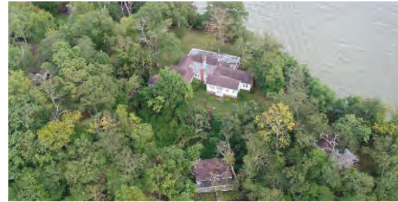
Former Residence Prior to Demolition: Aerial view of the abandoned house overlooking Loden Pond and the South River, later removed to restore the site's natural landscape and integrate it into Quiet Waters Park.
