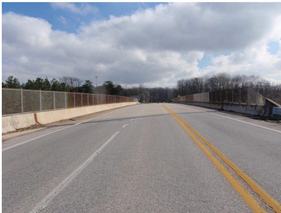
Figure 41: Sappington Station Crossing over MD 32 heading towards Burns Crossing Rd
