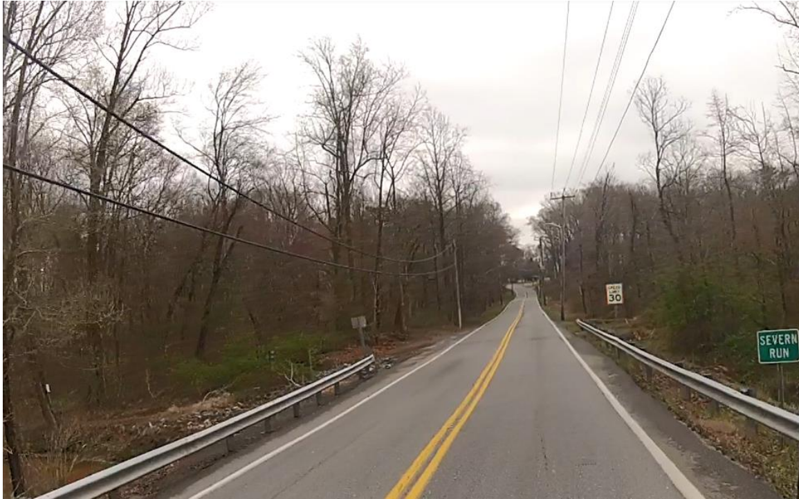
Figure 37: Burns Crossing Road, south of Old Mill Road has a narrow crossing over Severn Run
