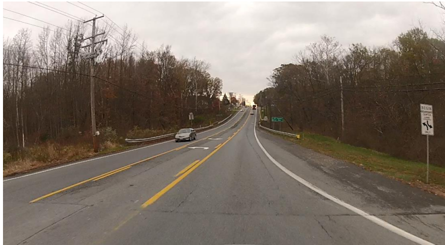
Figure 3: View of MD 170 (Telegraph Rd)
