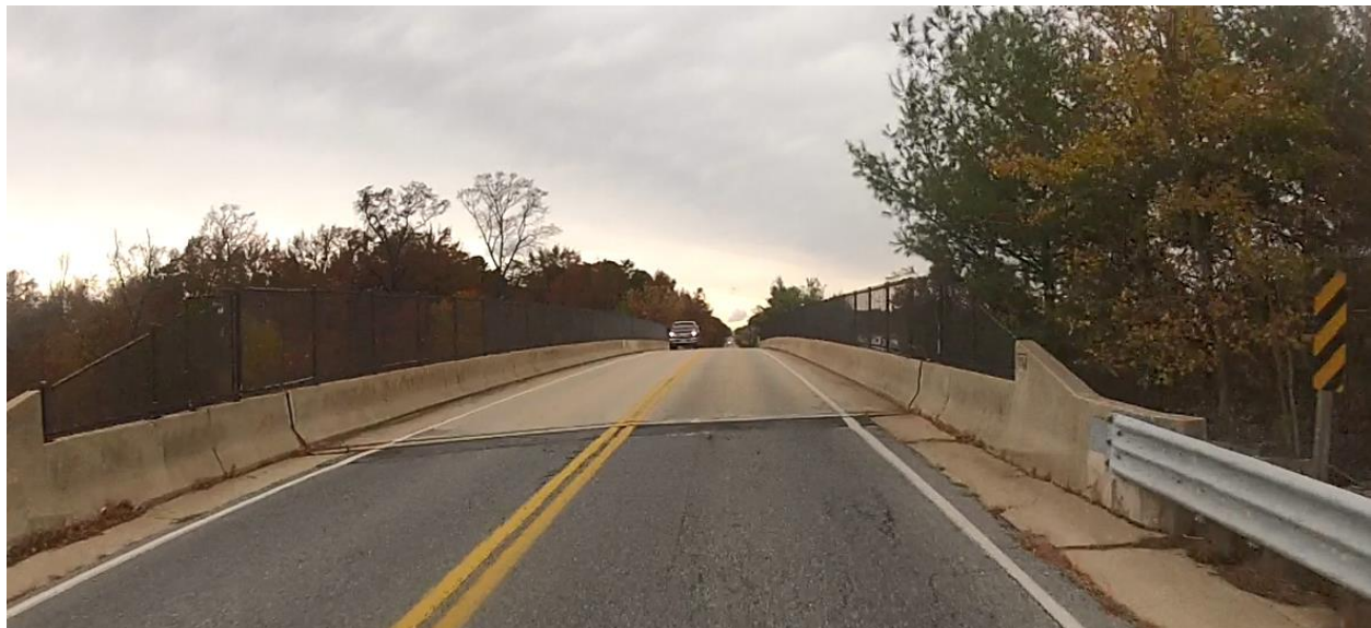
Figure 46: WB&A Road overpass over MD 100
