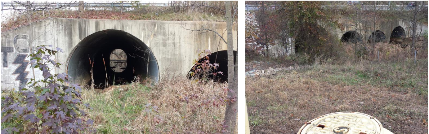
Figure 35: View of MD 32 Culverts looking north from an existing utility easement
