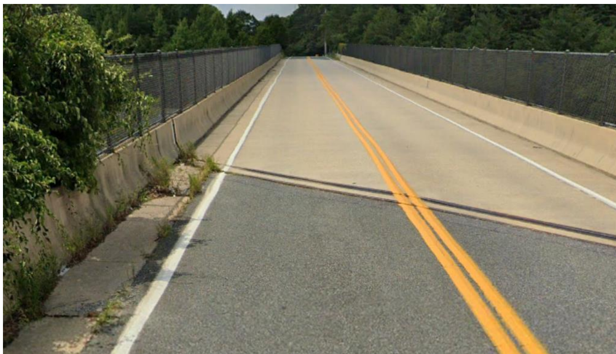
Figure 48: Queenstown Road overpass over MD 100
