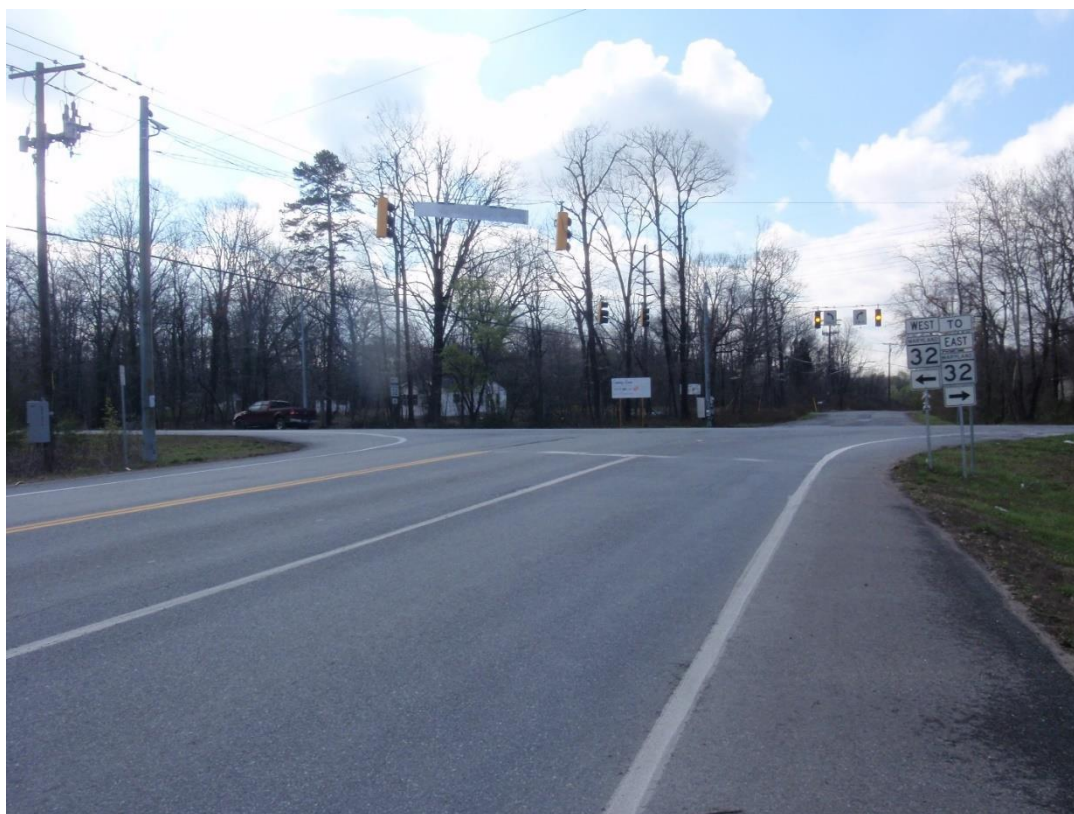
Figure 40: Burns Crossing Rd at Sappington Station Rd looking South
