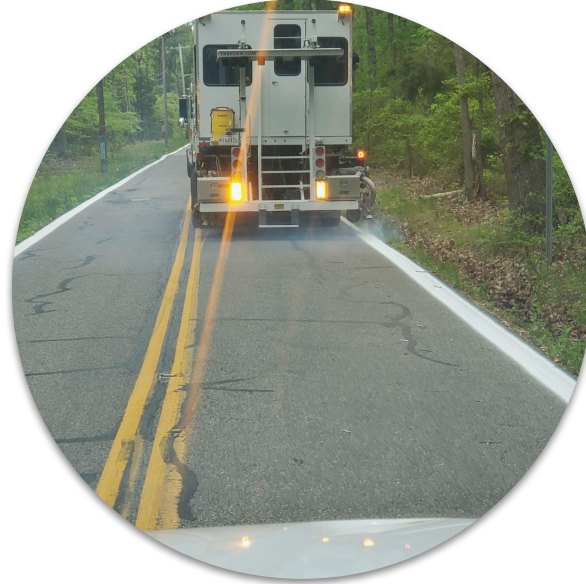
Long Line Installation
