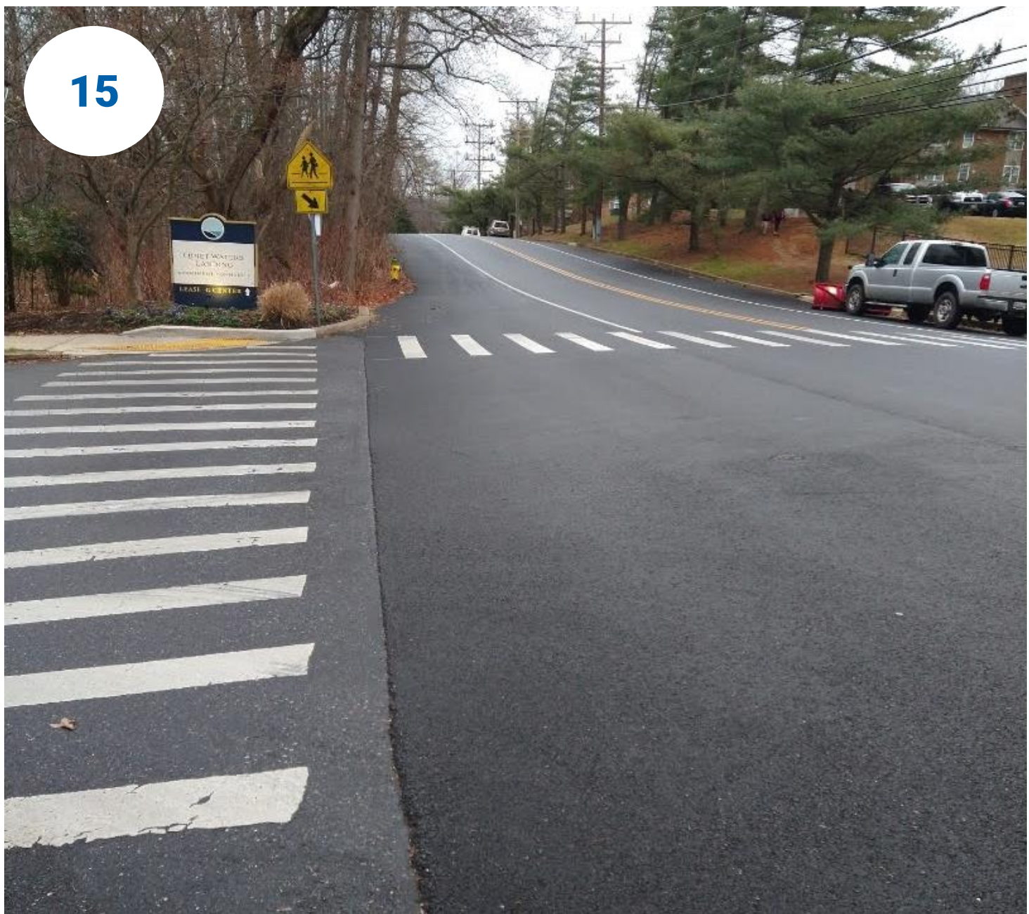
Bricin Street & Forest Hills Avenue
