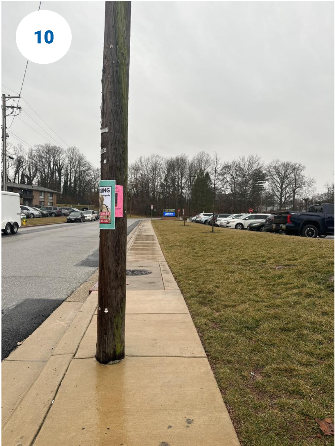
Sidewalk obstruction on Janwall Street
