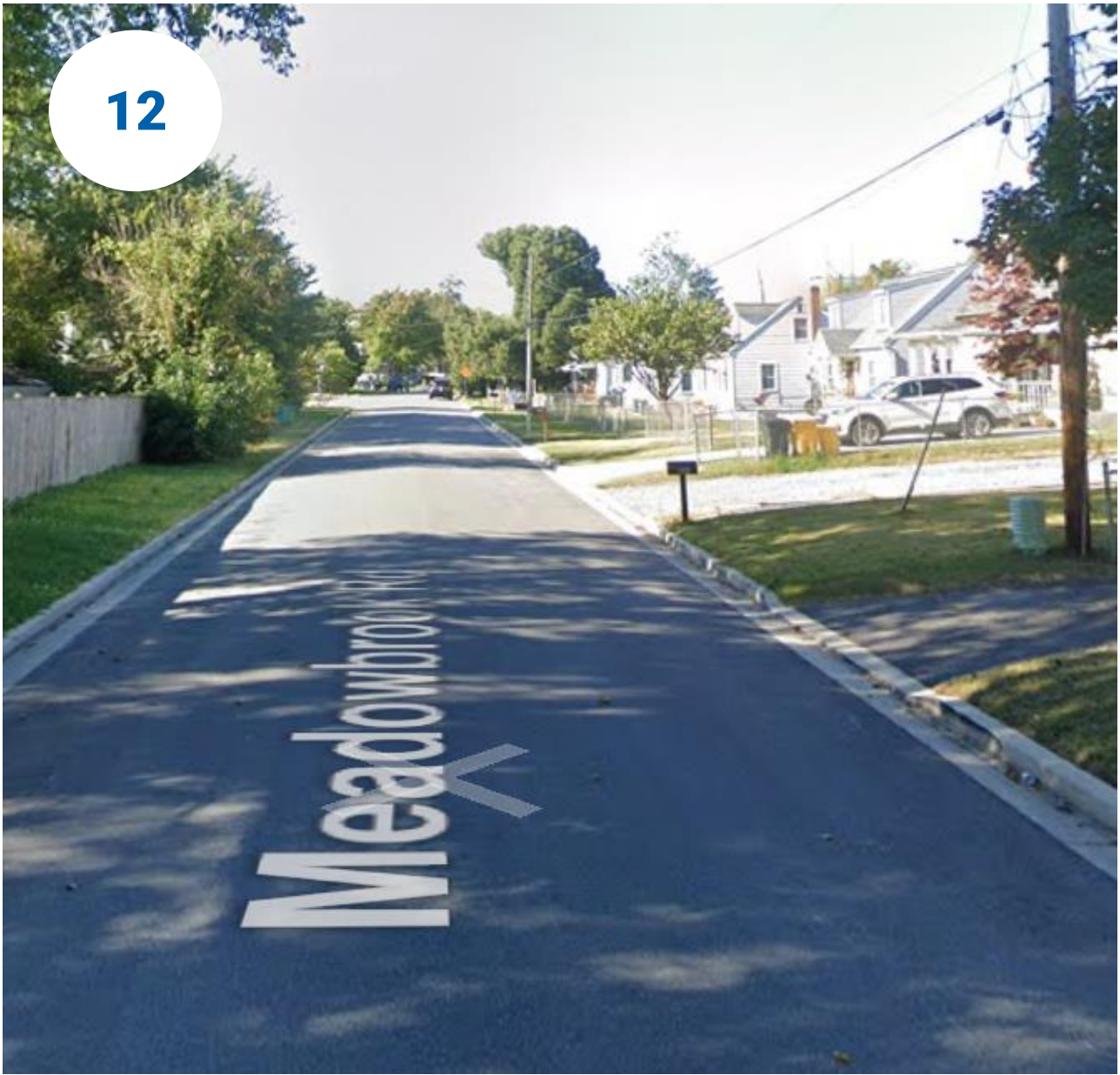
Meadowbrook Road, looking west
