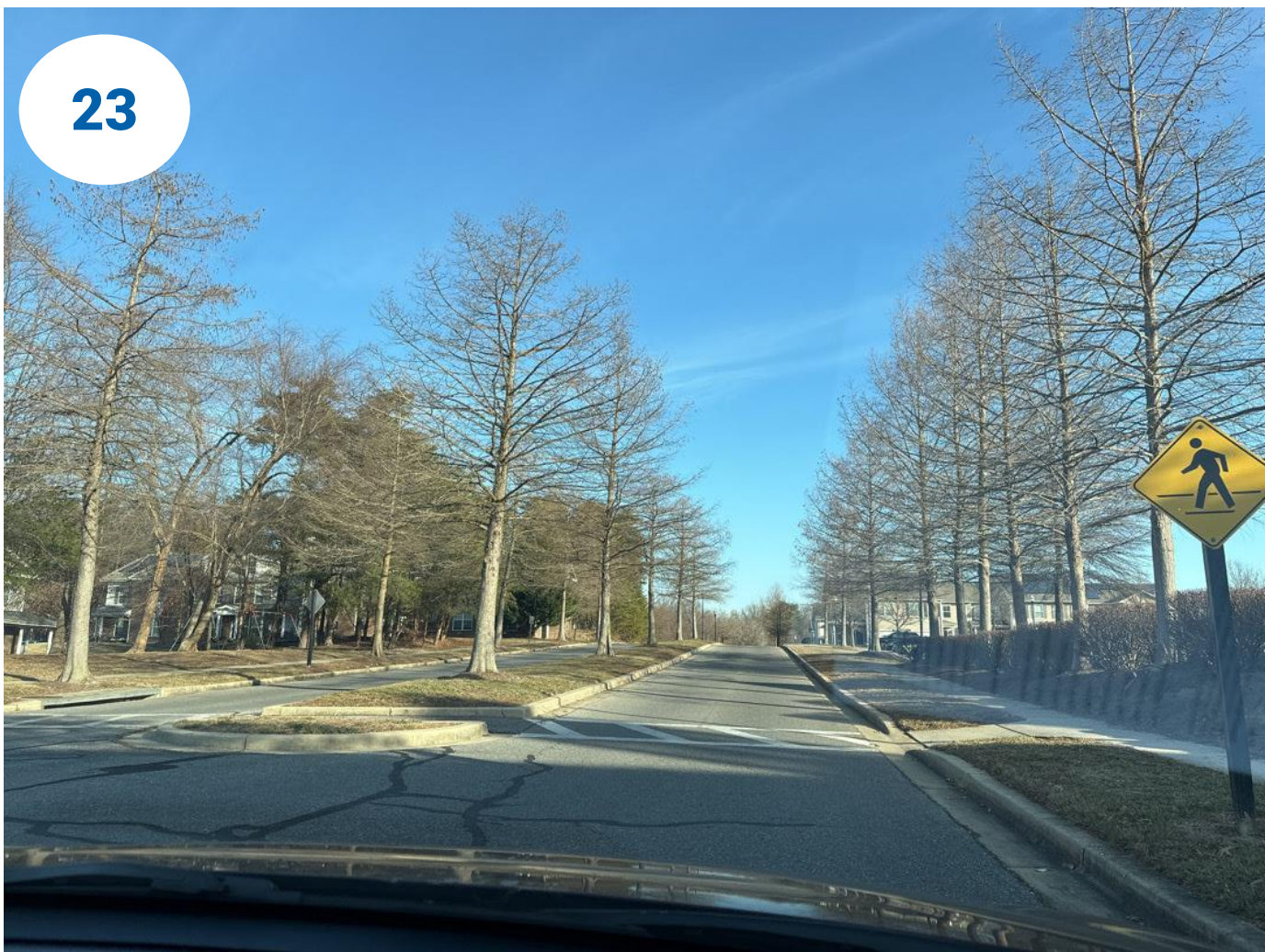
5 th Corps Road & 2 nd Corps Boulevard
