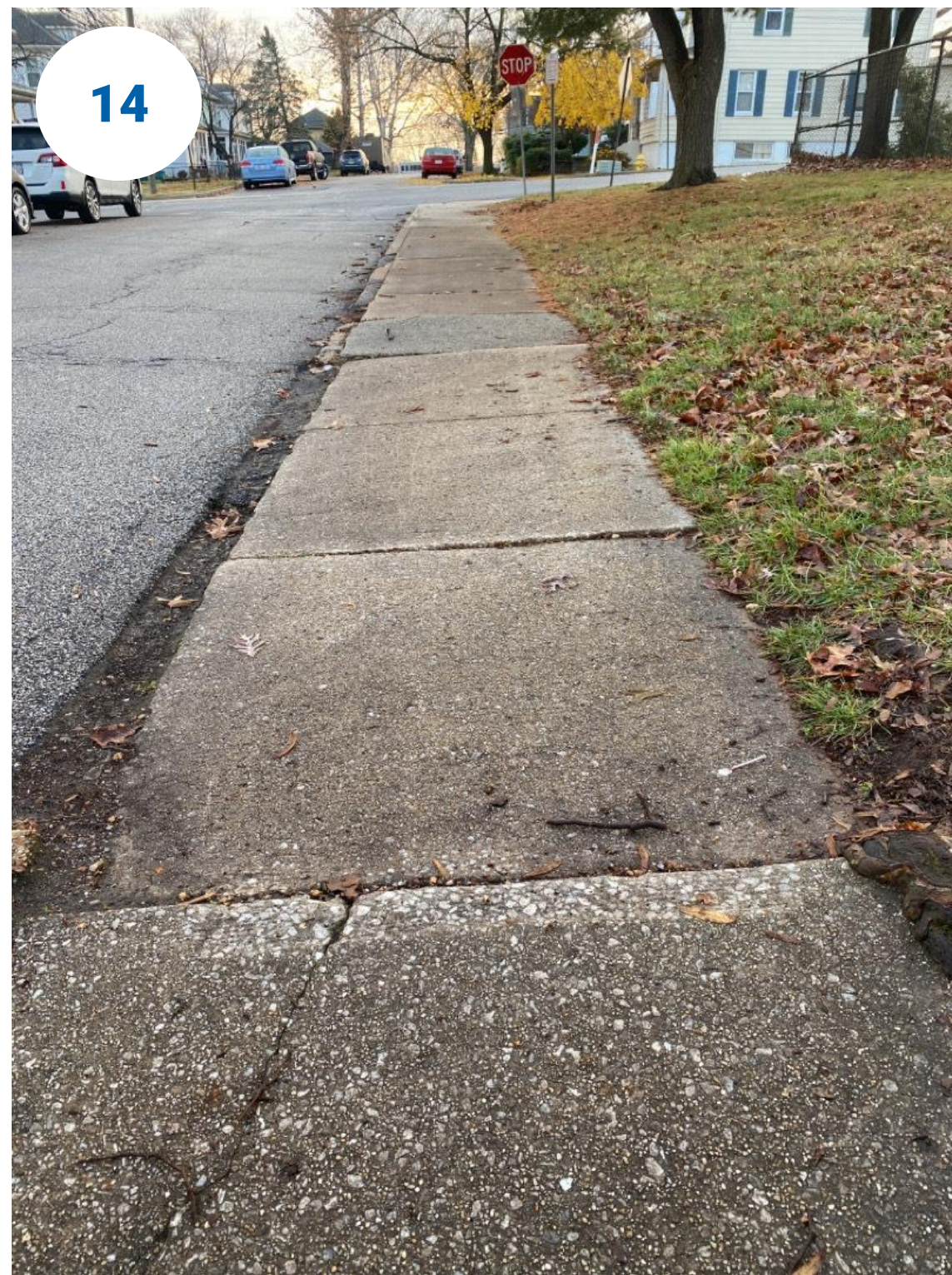
The existing sidewalk on 13 th Avenue
