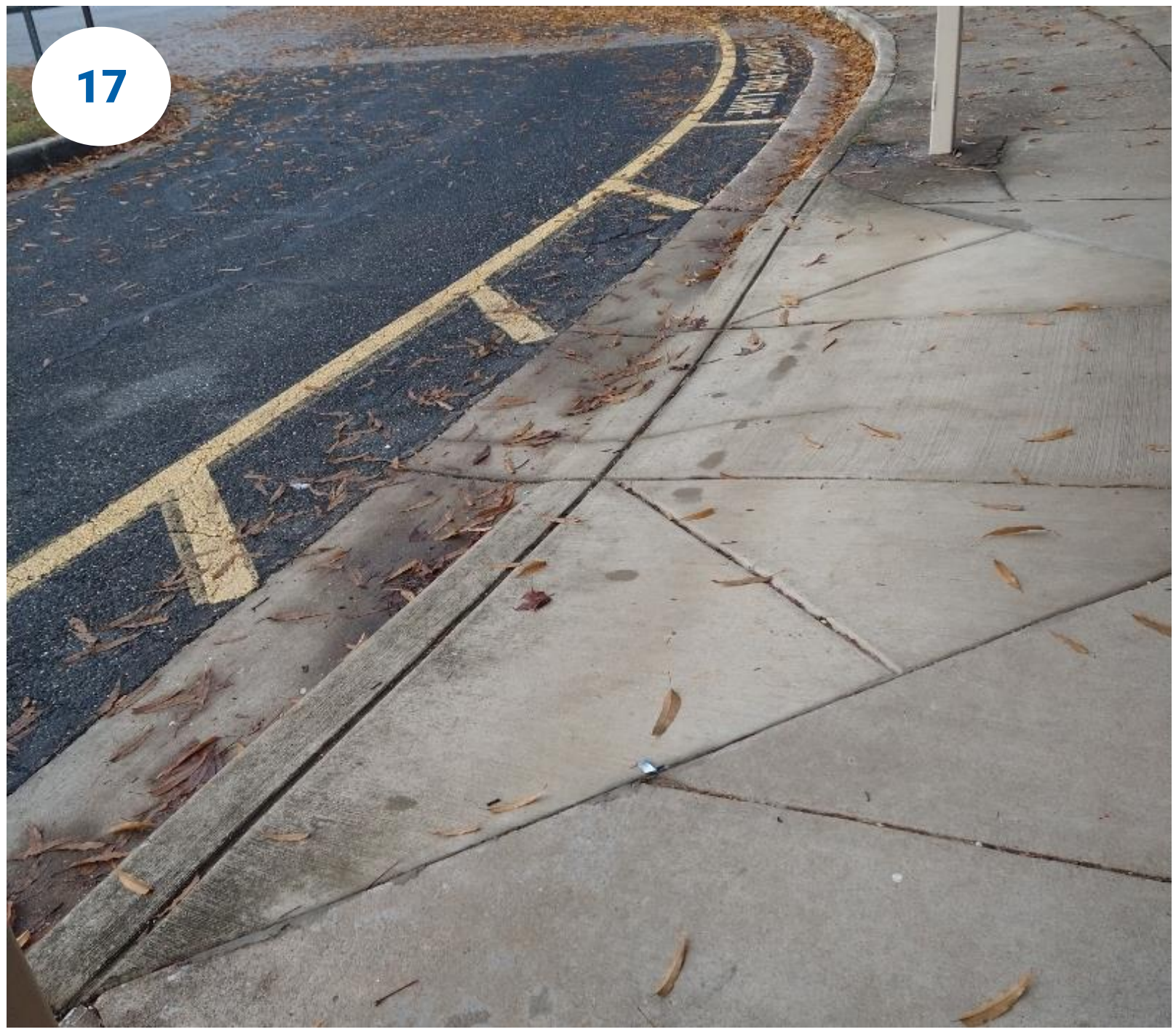
The curb ramp at bus drop off
