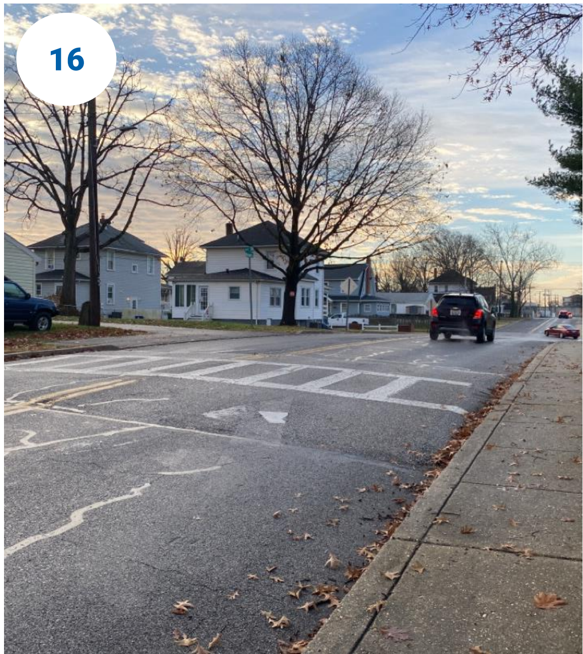
The existing speed hump on Morgan Road
