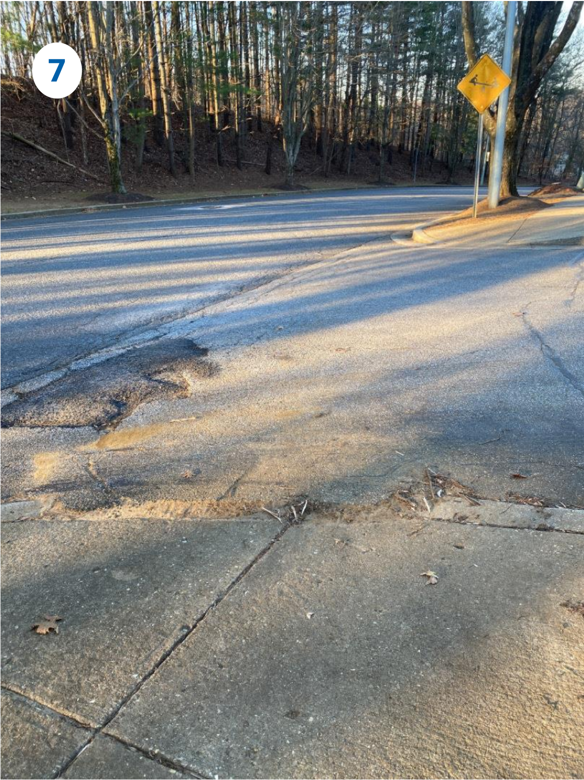
Crossing Palmwood Court at Greenhill Road
