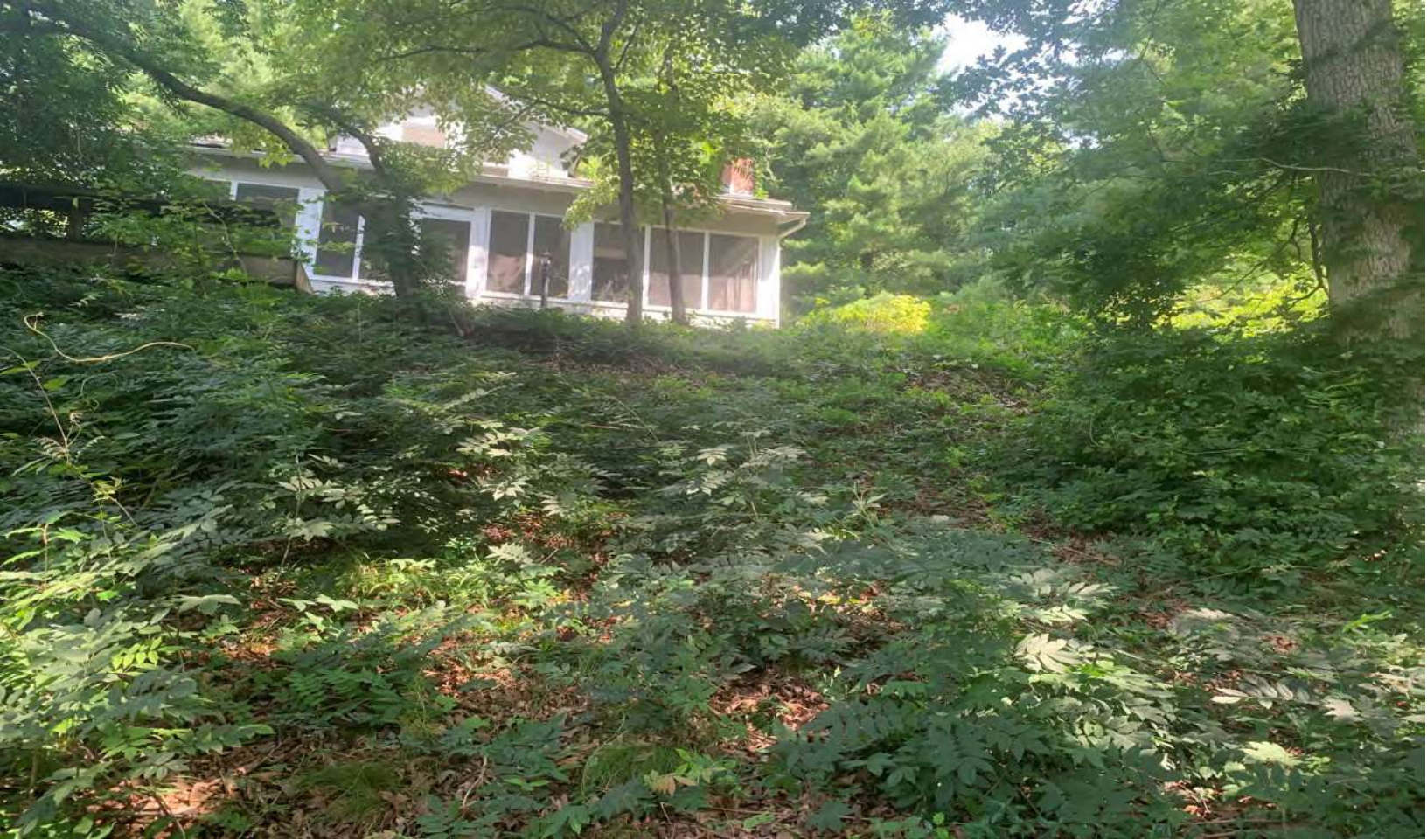
Photo #15 Looking North, Vegetatively Stabilized With Hardwood Trees, Shrubs & Ground Cover.
