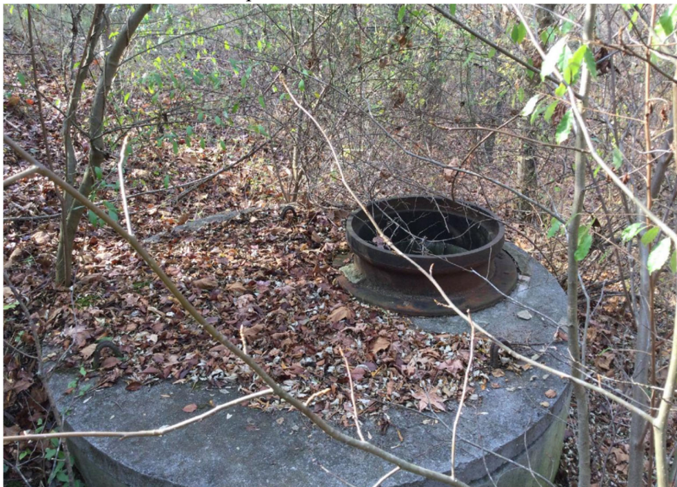
11/18/2024 Inspection- Upstream manhole, missing lid.
