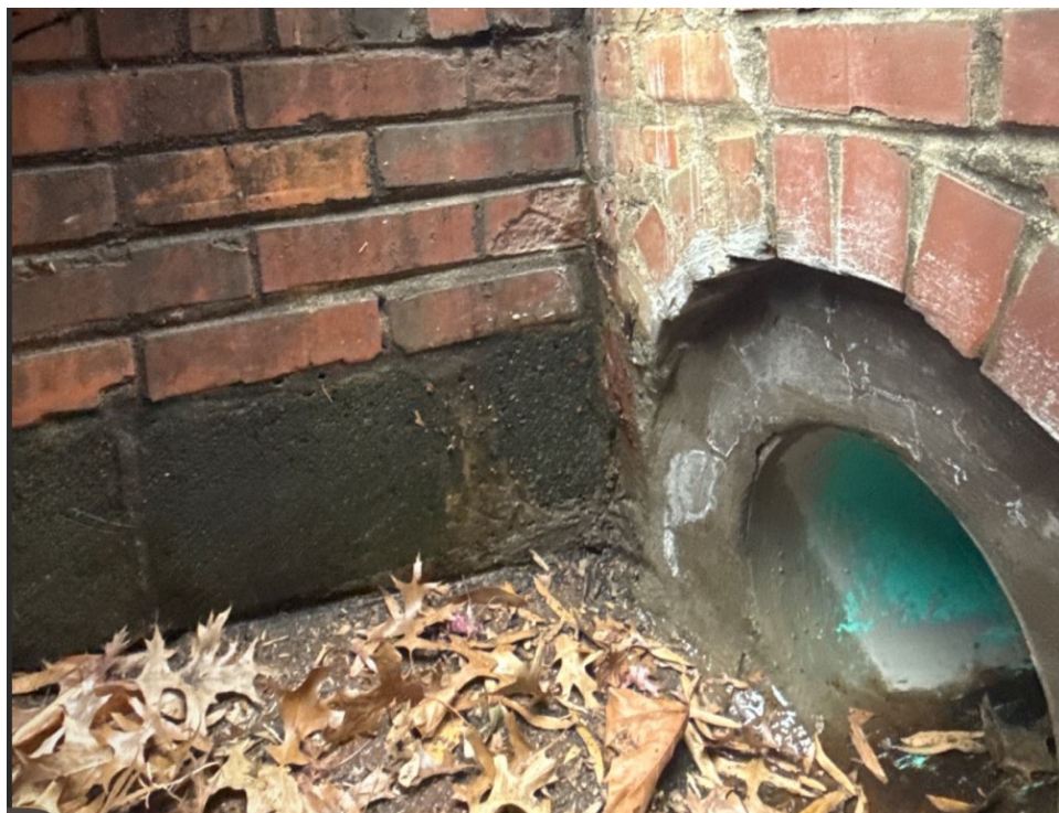
Interior of inlet connected to manhole with discharge source
