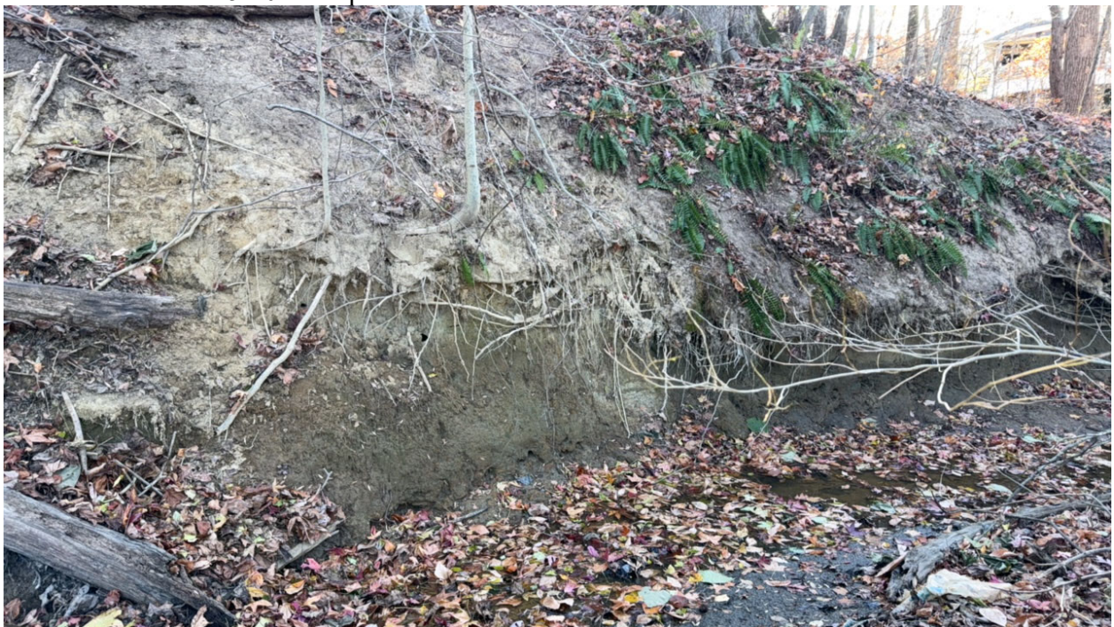
12/5/2024 Inspection- Severe downstream embankment erosion causing uprooting of trees.
