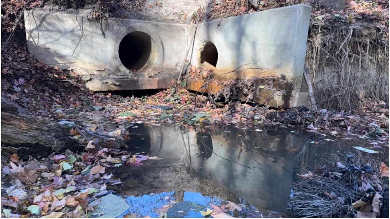
12/5/2024 Inspection- Upstream erosion is causing severe undermining and separation of the outfall structure from the surrounding hillside.
