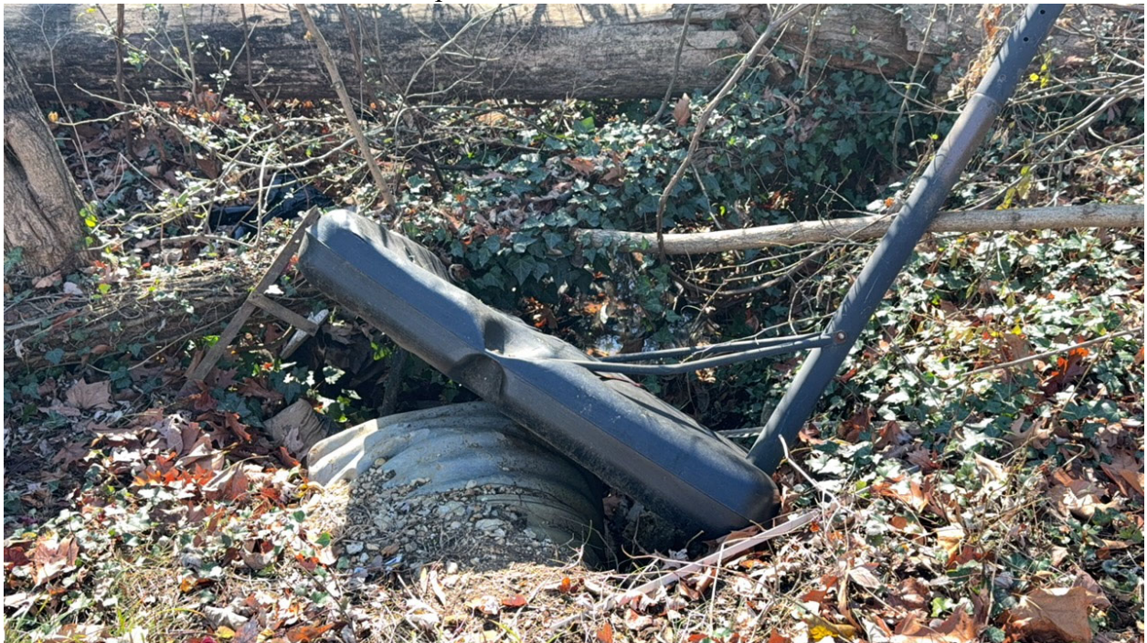
12/2/2024 Inspection- Downstream overview. Basketball hoop and debris blocking outfall channel.
