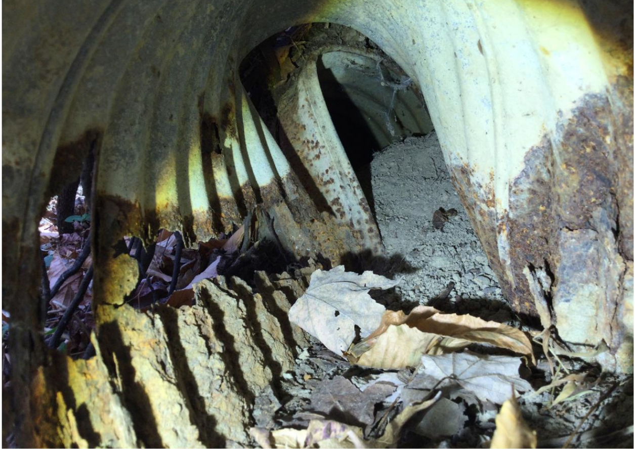
11/18/2024 Inspection - Secondary pipe is 25% filled with sediment and debris. Pipe is corroded and folding in on itself but may be abandoned.
