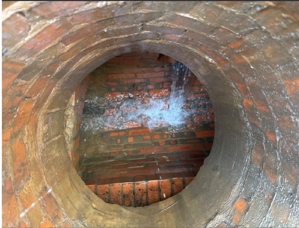
Interior of eighth upstream structure, source of discharge
