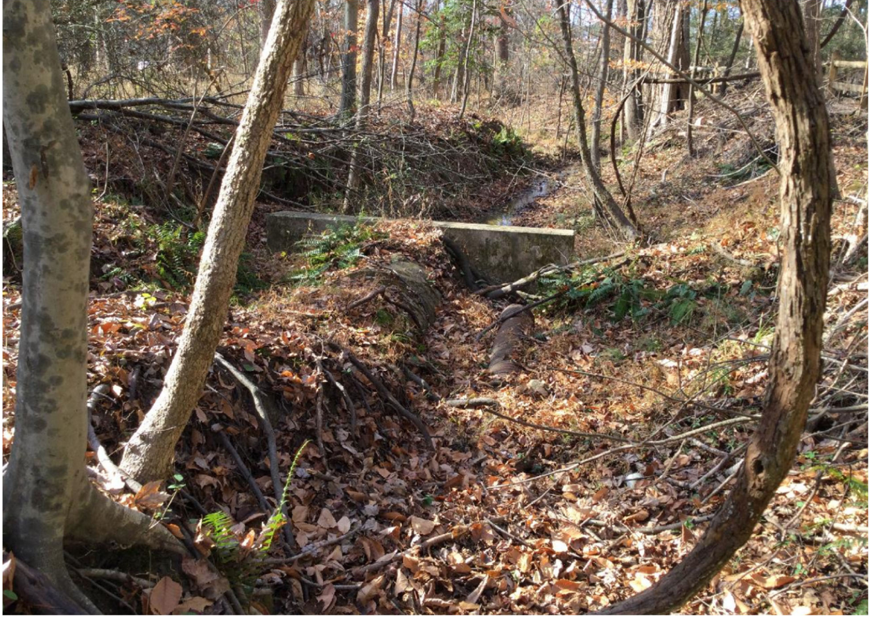
11/18/2024 Inspection - Erosion upstream of pipe causing pipe exposure.
