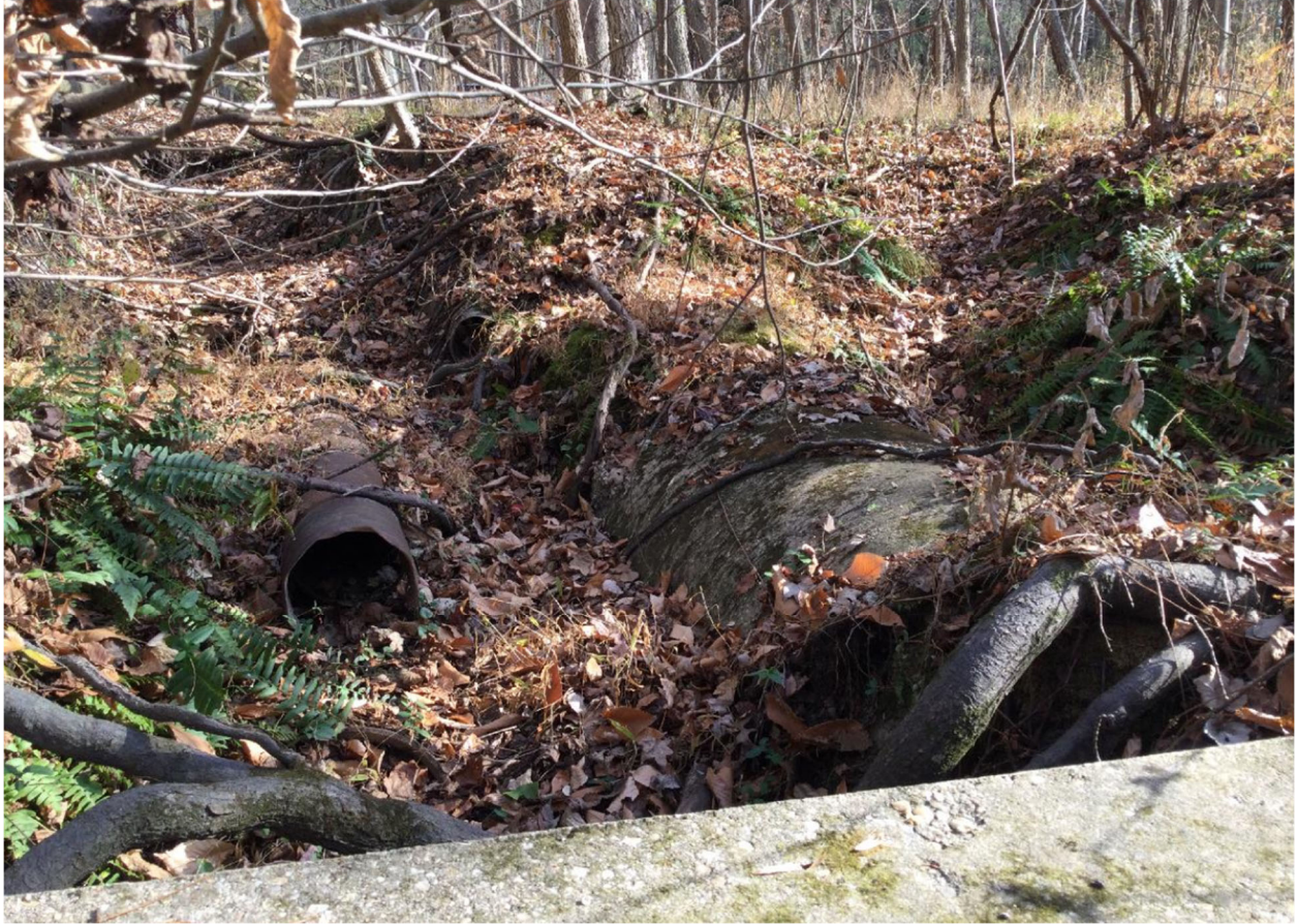
11/18/2024 Inspection - Erosion upstream of pipe causing pipe exposure. Secondary pipe is exposed and severely corroded but may be abandoned.
