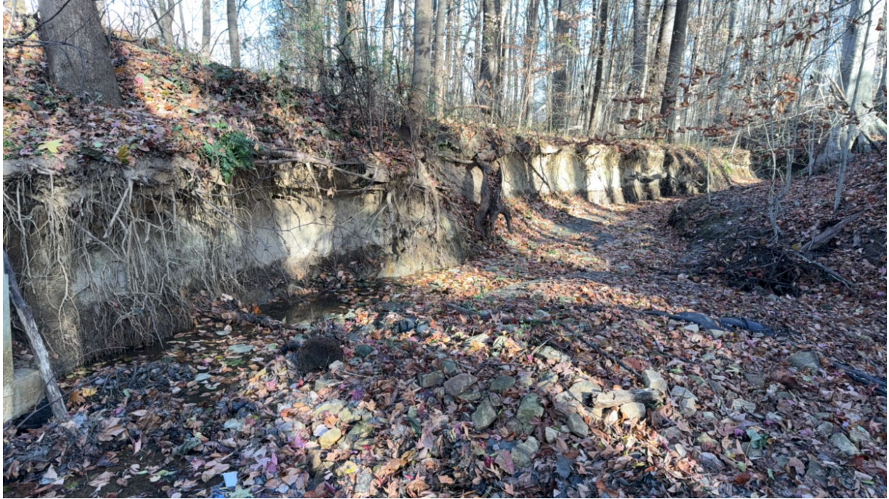
12/5/2024 Inspection- Severe downstream embankment erosion.
