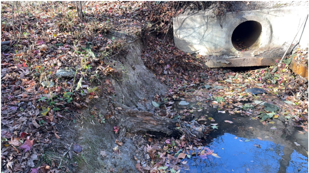
12/5/2024 Inspection- Downstream side slope erosion.
