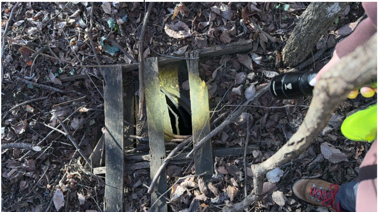
12/2/2024 Inspection- Upstream manhole, missing lid.
