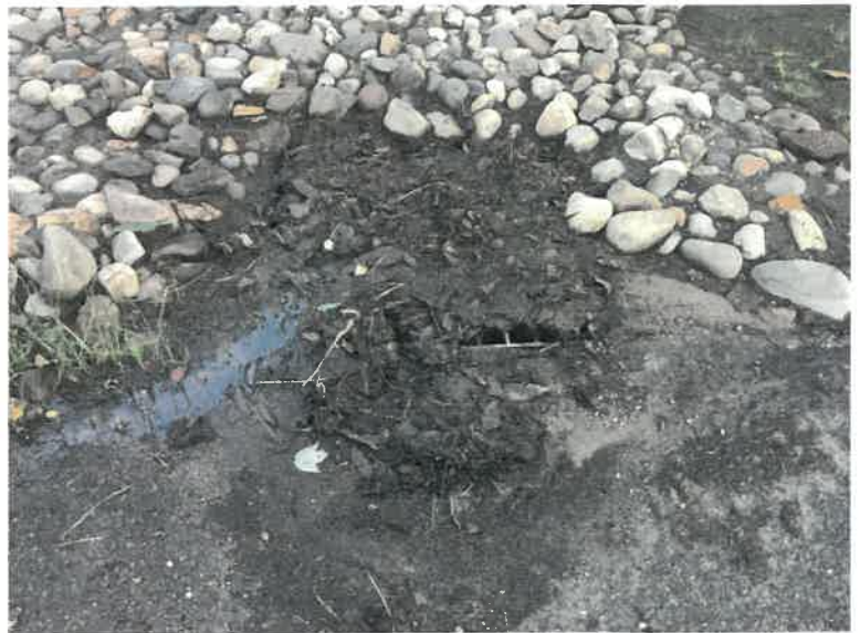
Grating over culvert between 8 & 10 Ridout Rd. blocked with mulch and debris following rainfall.
