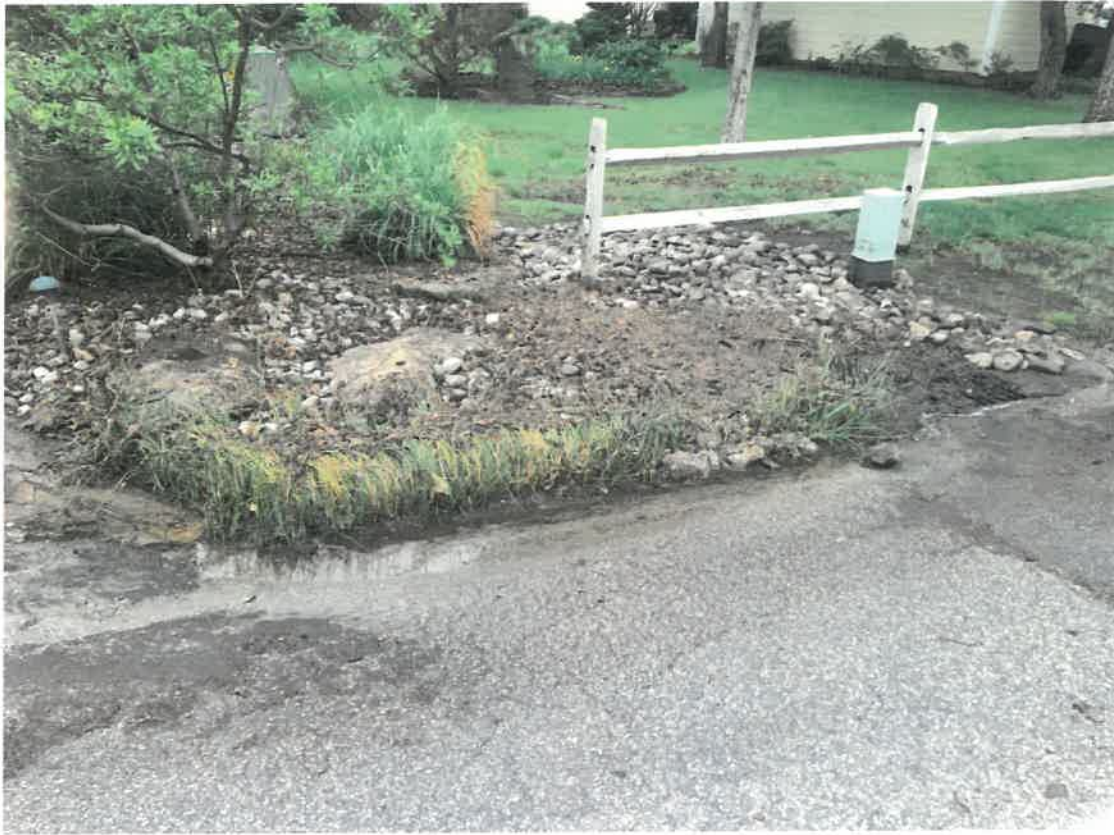
Grating (on the right) and surrounding area with mulch and debris from rain runoff
