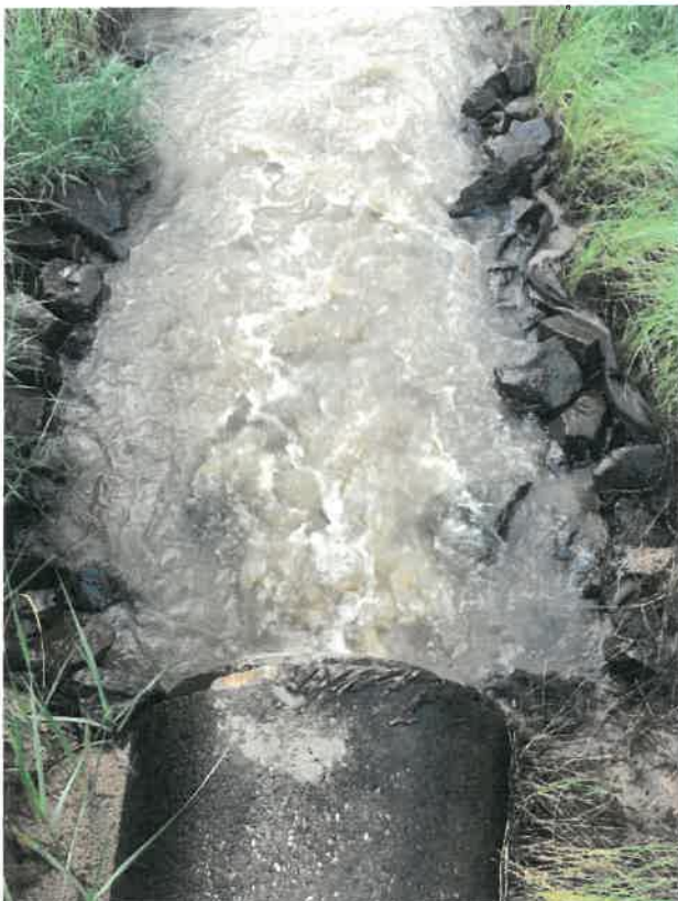
Silt laden discharge from Ridout Rd culvert into the Severn River.
