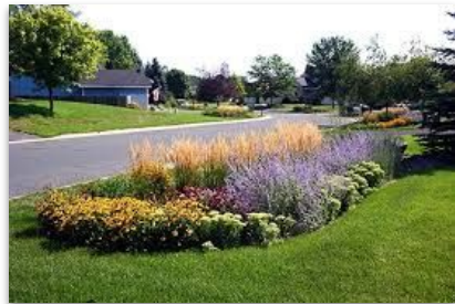
Landscaped Infiltration Garden
