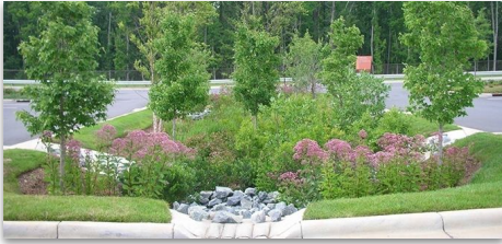
Micro-Bioretention 85% Coverage at Mature Growth
