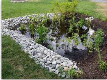
Standing Water (Silted in)
