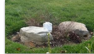
Plastic cap sticking out of the ground, not related to water or sewer
