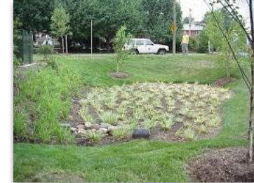
Micro-Bioretention Planting Plan Installed
