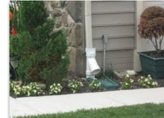
Downspout Connection to Underground Pipe
