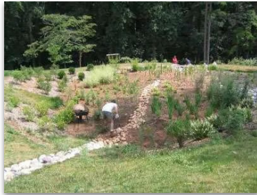
Micro-Bioretention Planting Plan Installed
