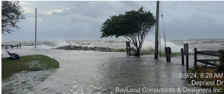
Photo 57 - Flooding and wave overtopping during Tropical Depression Debby
