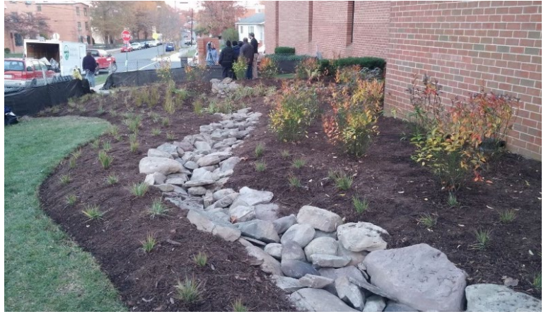
Photo 131 - Community-Built Bioswale at First Rock Baptist Church
