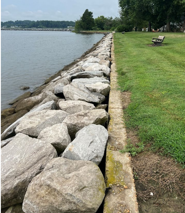
Photo 102 - Seawall with revetment along bay-fronting shoreline (Top of Seawall +6.5 feet NAVD88)
