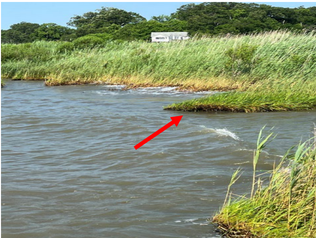
Photo 36 – Erosion of natural marsh edge south of Snug Harbor
