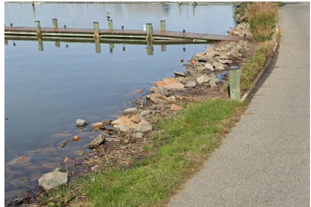
Photo 63 – Minimal stone protection along Chalk Point Road (Top of Stone +2.0' NAVD88)
