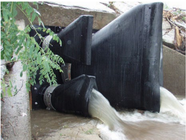
Photo 138 - Duckbill backflow prevention valve (source: Red Valve)
