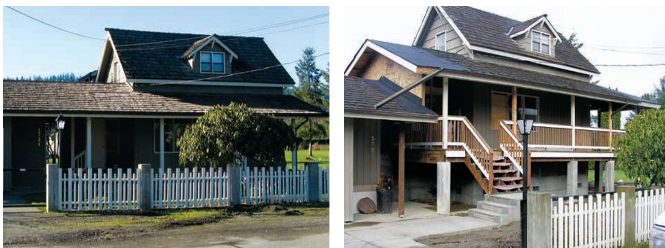
Photo 137 - Home Elevated 3 Feet in Snoqualmie, WA - Before (left) and After (right) 21
