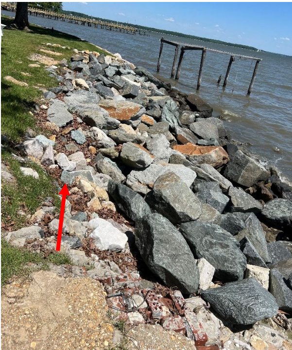
Photo 27 - Stone placed in washout areas
