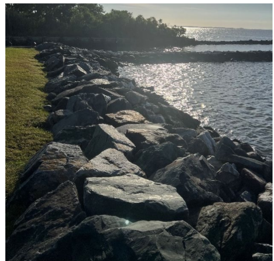
Photo 44 - Bay-facing revetment along community property near the marina entrance
