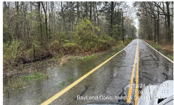
Photo 90 - Broadwater Road flooding during high tide event (April 12, 2024) Water level: +2.88' NAVD88 (or 2.2' above MHW)
