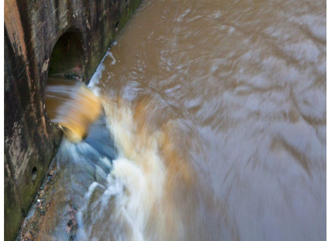
Photo 122 - Combined sewer systems discharge into waterbody
