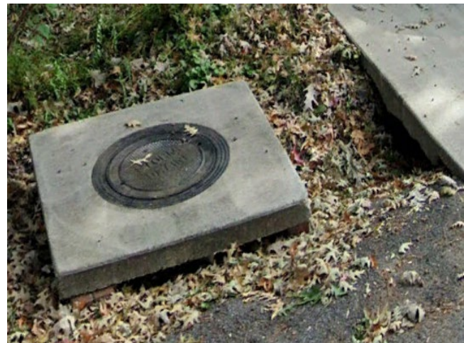
Photo 68 - Inlet filled with leaf litter
