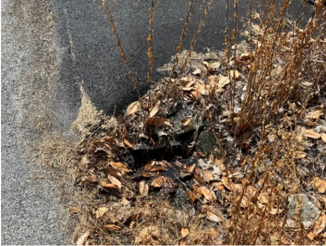
Photo 38 – Blocked culvert
