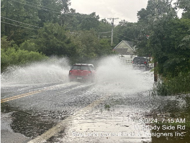
Photo 15 - Overtopping of Shady Side Road near St. Matthews United Methodist Church Water level: +3.53' NAVD88 (or 2.87' above MHW)
