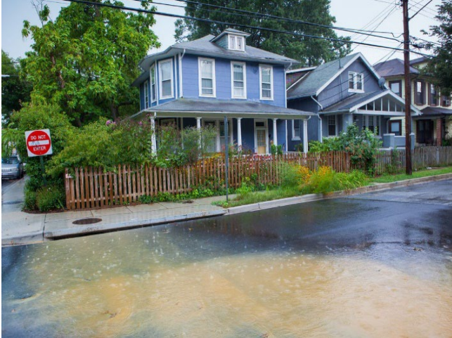
Photo 121 - Combined sewer system backs up into residential streets in Washington D.C.
