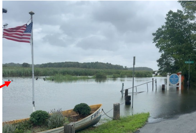
Photo 76 - Franklin Manor Boat Club boat ramp and parking area during Tropical Depression Debby (August 9, 2024) Water level: +3.66 NAVD88 (or 3' above MHW)
