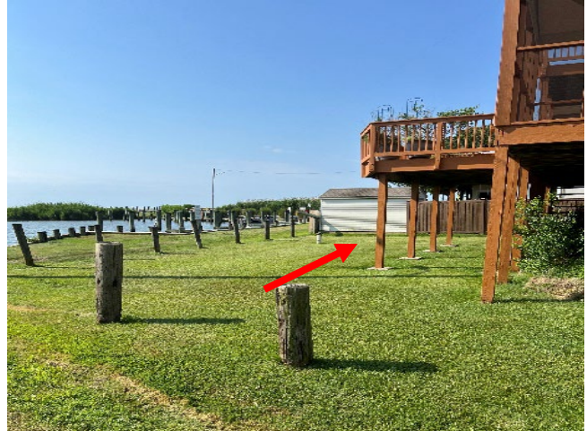
Photo 33 - Elevated home behind marina bulkhead
