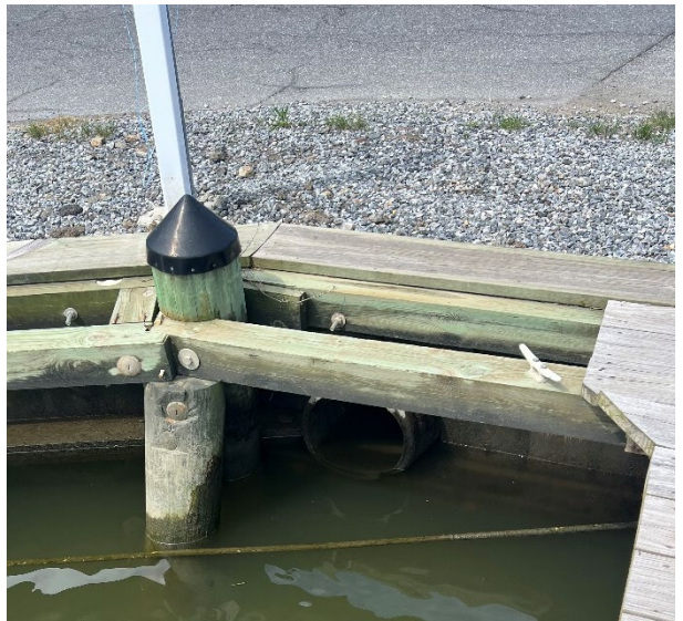
Photo 50 - Partially submerged tidal outfall at the Cedarhurst Marina
