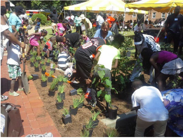
Photo 130 - Volunteers installing green infrastructure project sponsored by RiverSmart Communities Program
