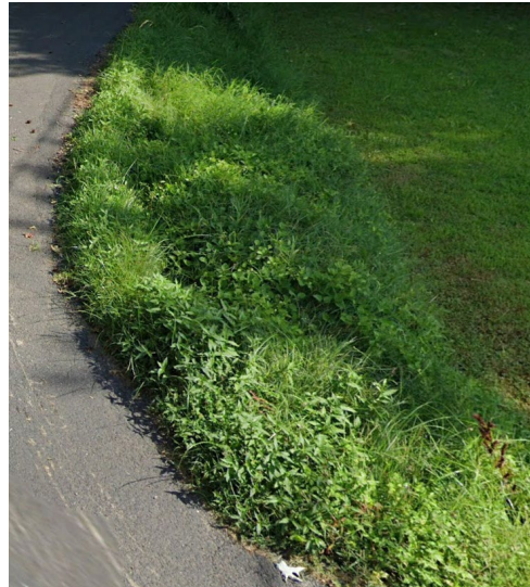
Photo 22 - Overgrown swale
