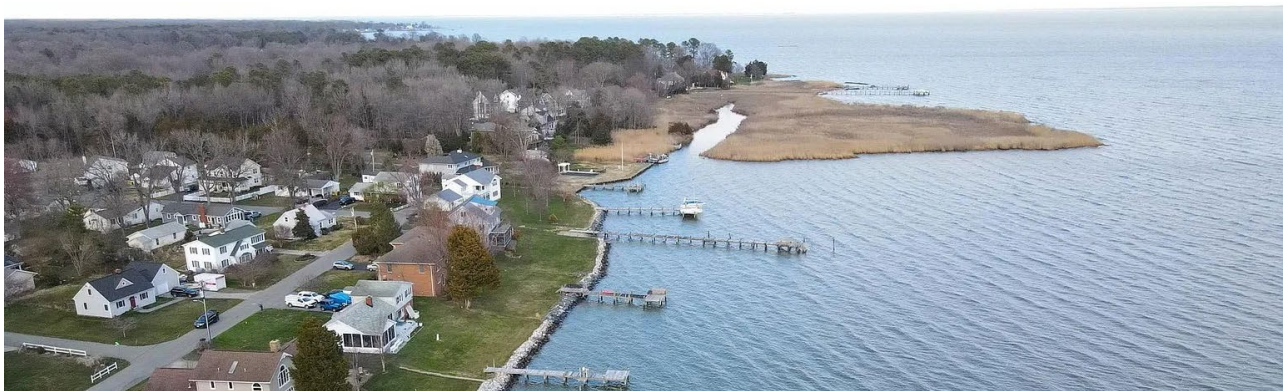
Photo 92 - Bay-facing shoreline protected by stone revetments and natural wetlands.
