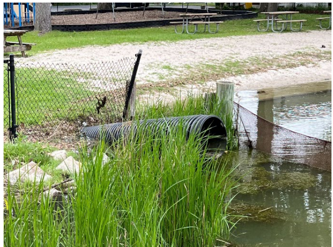
Photo 12 - Outfall at Community Park Water level: +2.09' NAVD88 (or 1.43' above MHW)
