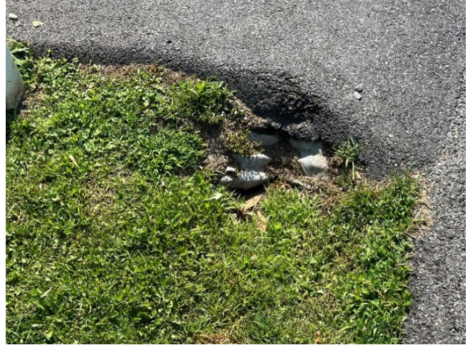
Photo 39 – Crushed culvert
