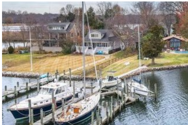
Photo 64 - Private properties armored with revetments along Chalk Point's shoreline
