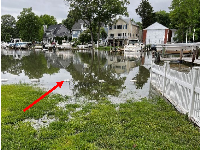
Photo 9 – Bulkhead submerged at high tide (Top of Bulkhead between +2' and +2.5' NAVD88)
