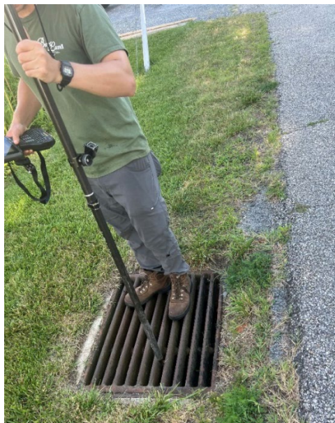
Photo 5 – Surveying inlet elevation and location
