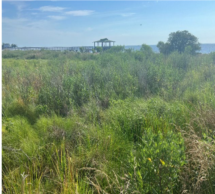
Photo 45 - Non-tidal marsh protected by stone revetment between Chesapeake Avenue and the bay (Top of Stone +4.5' NAVD88; Marsh Elevation +1.5' to +3.0' NAVD88)
