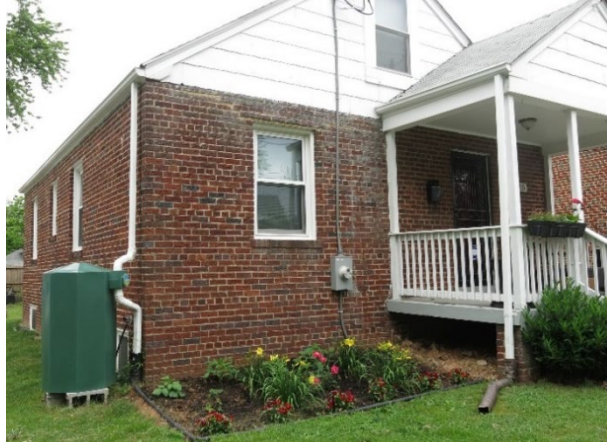
Photo 126 - Rain Barrel install supported by RiverSmart
