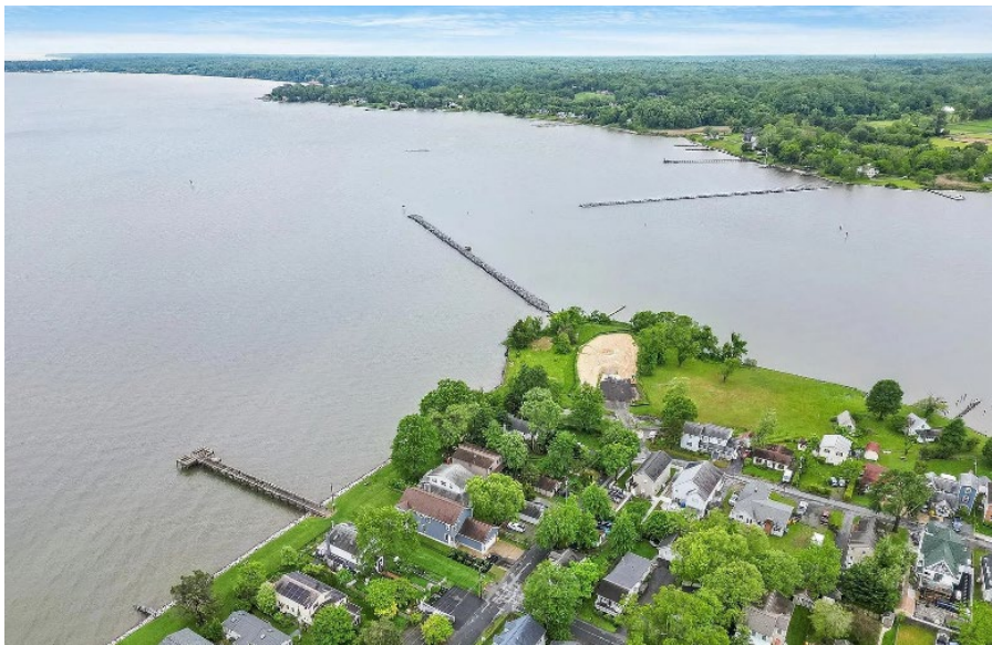
Photo 104 - SSW aerial view of southern tip of the community and stone jetties at the entrance to Rockhold Creek (Top of Stone +6.0 feet NAVD88)
