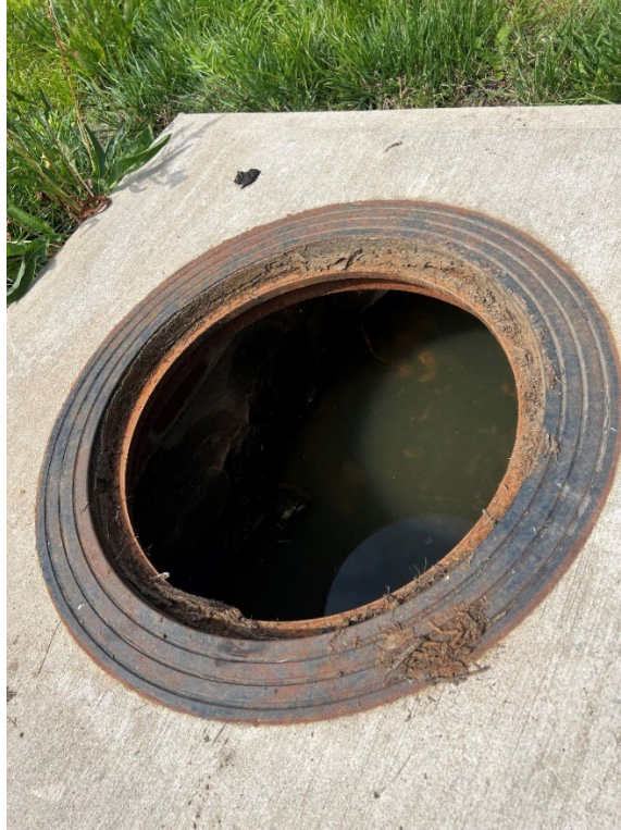
Photo 51 - Flooded inlet approaching low tide Water level: +0.03' NAVD88 (or 0.63 below MHW)
