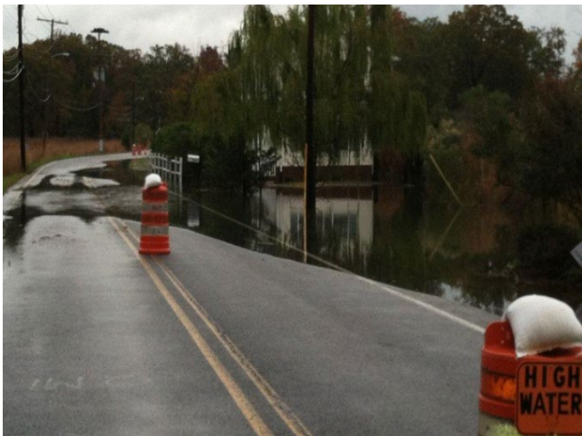
Photo 113 - Flooding at Bay Avenue during Hurricane Sandy (2012) – Photo from northbeachmd.org
