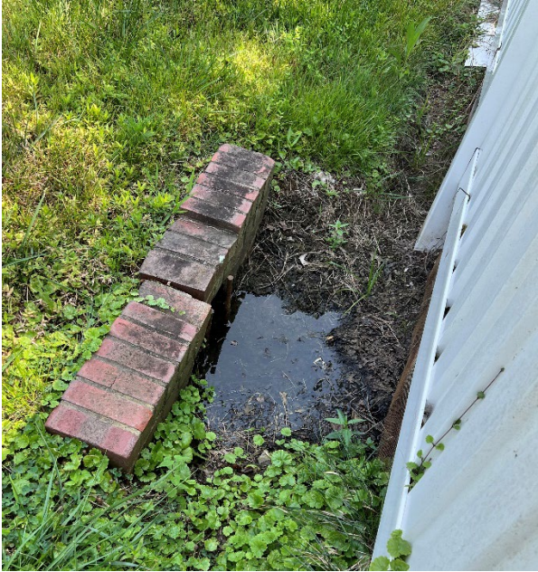
Photo 80 - Roadway culvert at Gwynne Avenue and Exeter Street backwatered during "Sunny Day" flooding Water level: +1.5' NAVD88 (or 0.8' above MHW)
