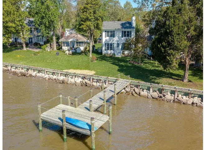
Photo 98 - Standard residential shoreline protection along bay-facing shoreline in Masons Beach (Top of Bulkhead +7.0 feet NAVD88)
