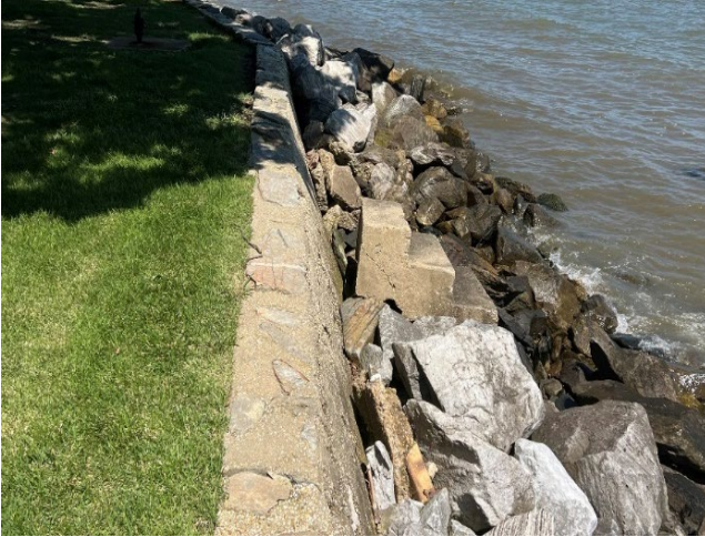
Photo 25 - Seawall with stone protection (Top of Wall +5' NAVD88)
