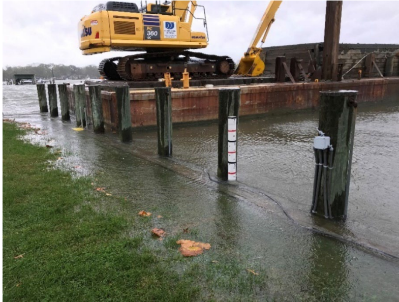
Photo 18 - CYC flooding during storm (October 29,2021) Water level: +3.45' NAVD88 (or 2.79' above MHW)
