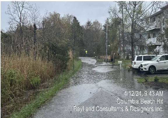
Photo 55 - Columbia Beach Road during high tide flooding in April Water level: +3.22' NAVD88 (or 2.6' above MHW)
