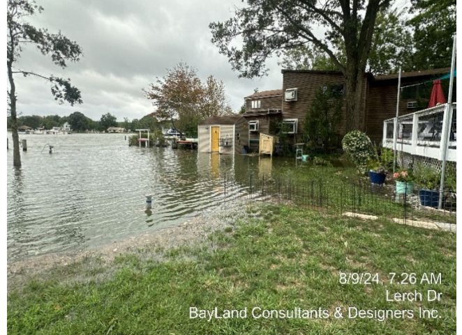
Photo 16 - Floodwaters encroaching into residential property and infrastructure Water level: +3.6' NAVD88 (or 2.94' above MHW)
