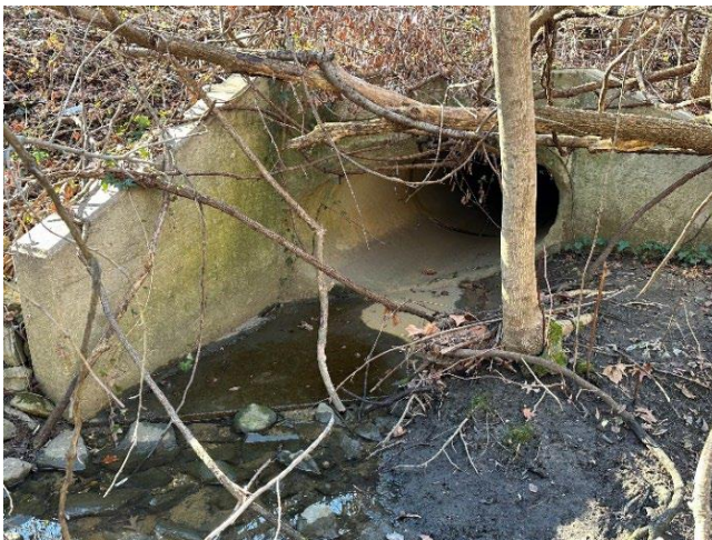
Photo 1 – 60-inch x 38-inch RCCP elliptical outfall
