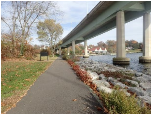
Photo 60 – Paved path along western edge of park under Naval Academy Bridge
