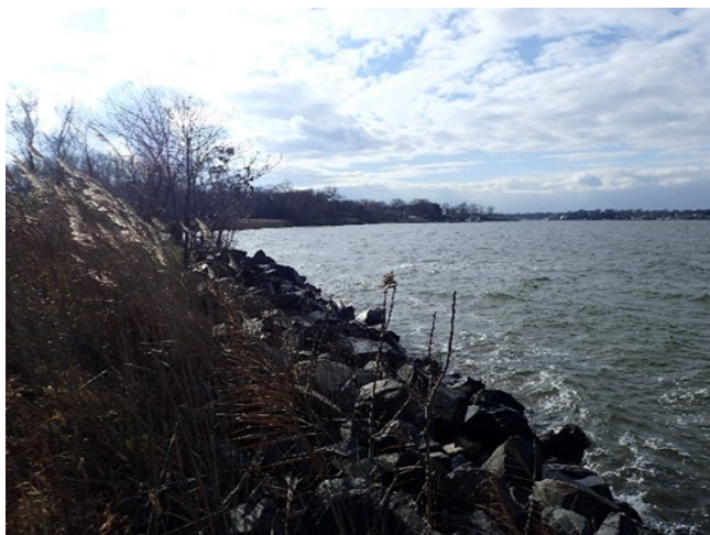
Photo 33 – Stone revetment along northern point
