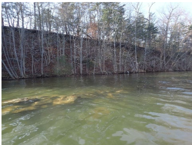
Photo 3 – Submerged sills along Severn River shoreline
