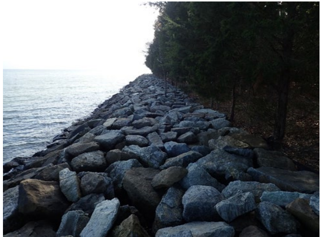
Photo 53 – Revetment along Chesapeake Bay
