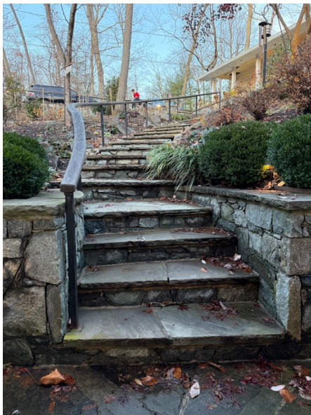
Looking up from front door to garage: More than 15 ft drop over 23 steps, which are steep and dangerous. Person at top of steps is barely visible.
