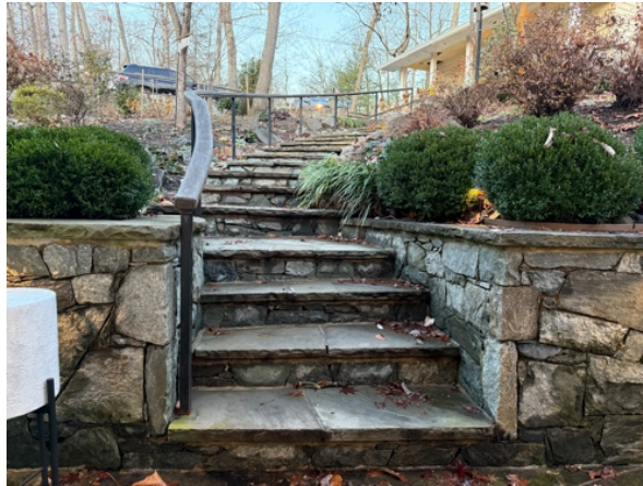
Looking up from front door to garage: More than 15 ft drop over 23 steps, which are steep and dangerous
