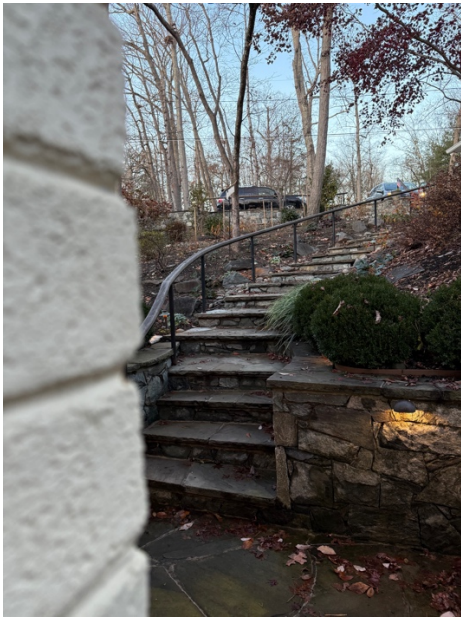
Looking up from front door to garage: More than 15 ft drop over 23 steps, which are steep and dangerous
