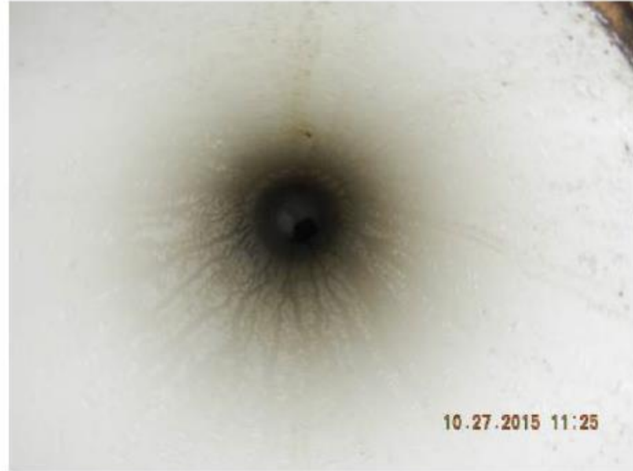
View inside the observation well, clear of water and sediment.
