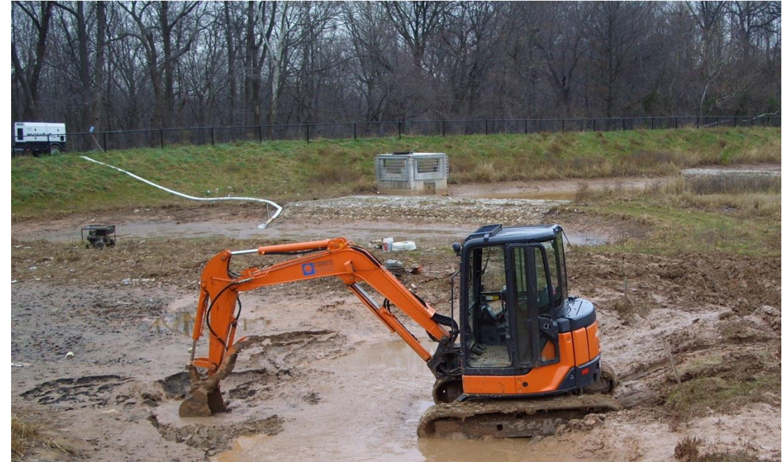
Chesapeake Bay Stormwater Network
