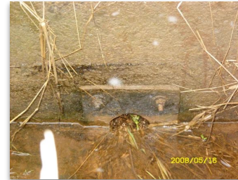
Blocked Low-Flow Orifice
