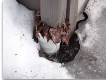
Clogged Downspouts, Disconnection from Ground Connector
