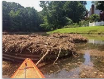
Trash/Debris on Riser
