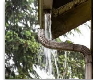
Disconnected Roof Gutter
