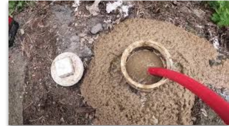
Blocked Underdrain, Cleanout, Observation Well
