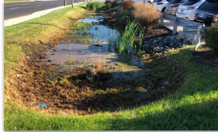
Standing Water (Blocked Underdrain)
