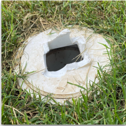
Broken, Buried, or Missing Cleanout/Observation Well Caps
