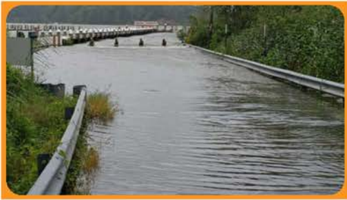
Edgewater, MD Flooding August 2024
