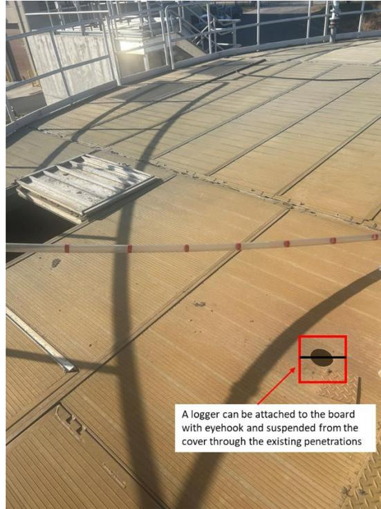
**Figure 2-6 Gravity sludge thickener PPM monitor location**
