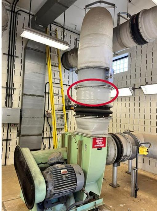
**Figure 2-7 Proposed H<sub>2</sub>S monitoring location at the aeration blower facility**
