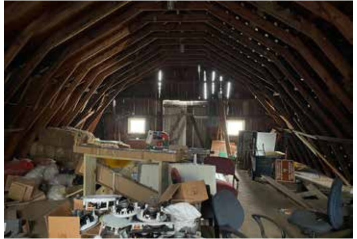
Figure 17. Second floor of barn is used for storage and has visible exposure to the outside
