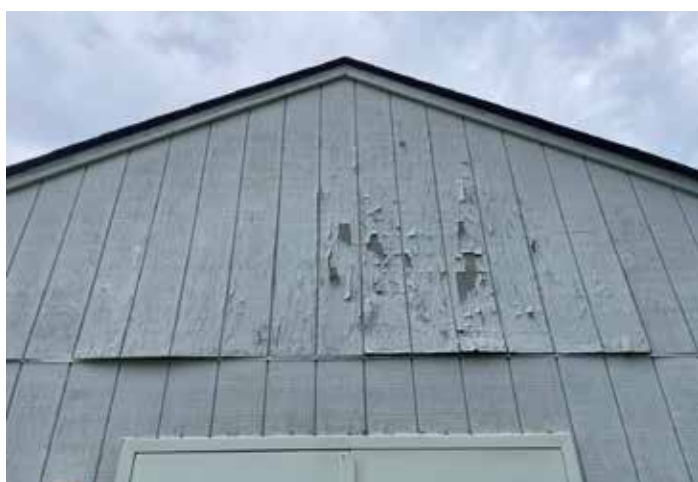
Figure 24. Chipping paint on front of greenhouse
