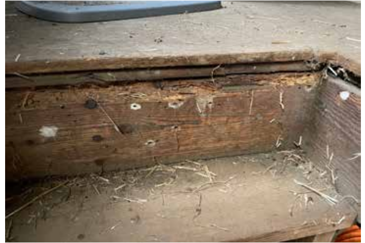
Figure 20. Second floor landing has visible damage
