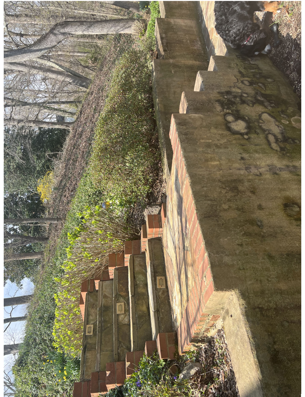
Existing Exterior Staircase - Uneven Riser Heights
