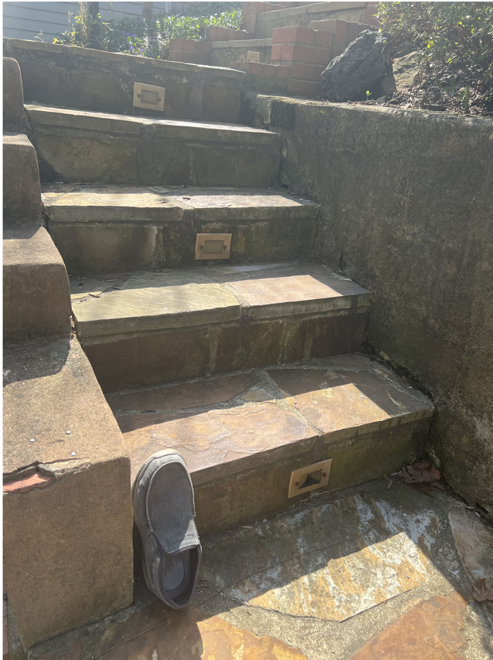
Existing Exterior Staircase - Uneven Riser Heights
