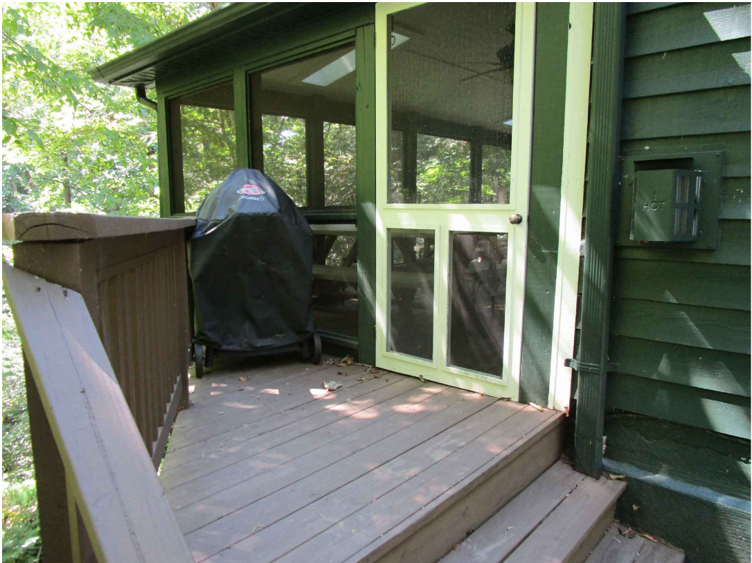
Existing Lower Level Screened Porch (Southern Facade)
