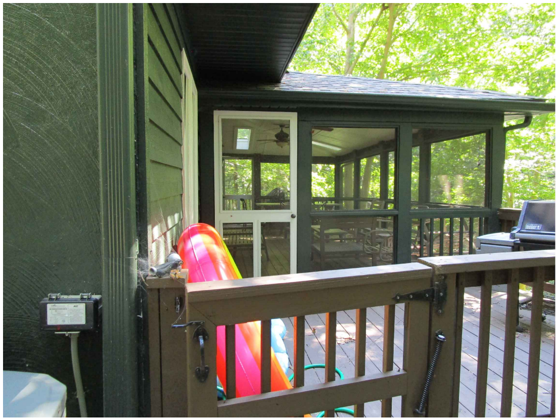
Existing Lower Level Screened Porch (Northern Facade)
