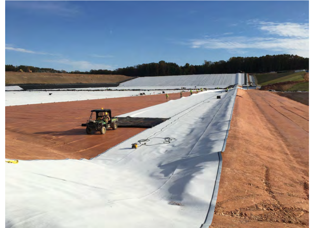
Geosynthetic Bottom Liner Deployment - Subcell 9.2
