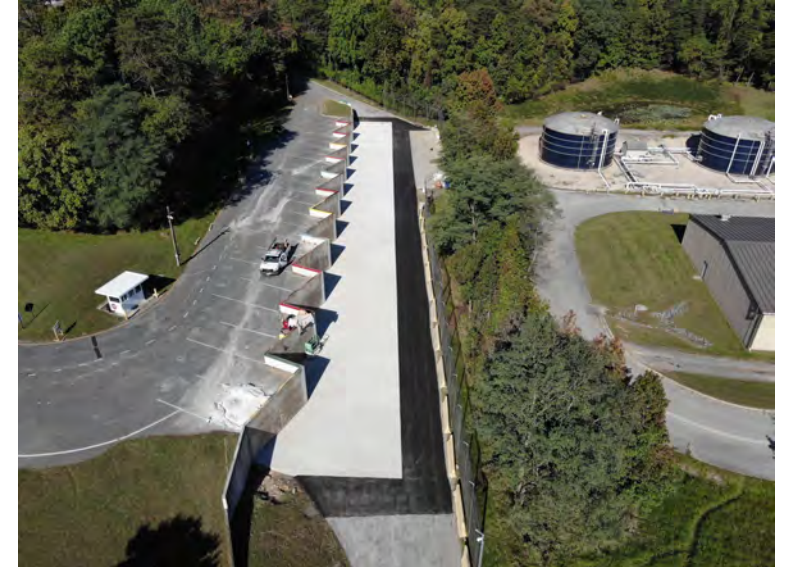
Central Recycling Center Lower Recycling Wall Renovation - 2023
