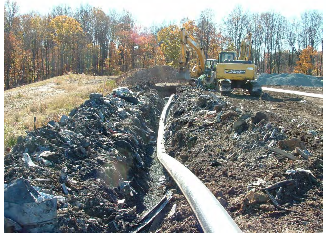
Temporary Gas Collection System Install Subcell 9.1
