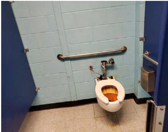
Women's Bathroom Water Closet
