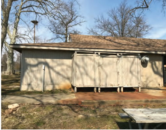
Exterior of Roof
