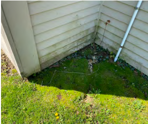
Exterior detail view
