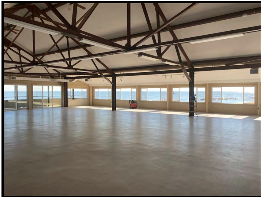
6. Hall banquet room interior
