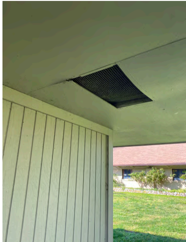
Siding and Roof Vent
