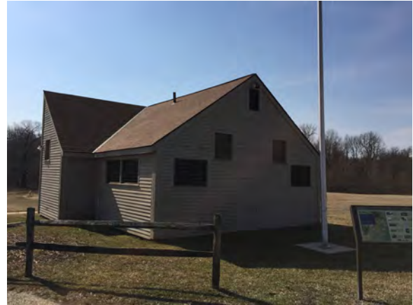
Exterior View of Stick-Framed Roof
