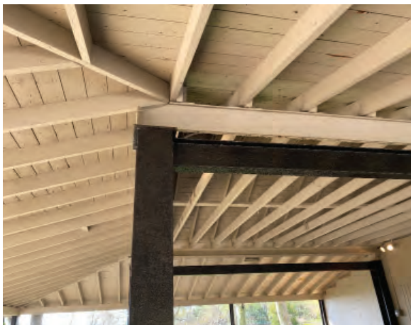
Wood Rafters with Steel Columns and Beams
