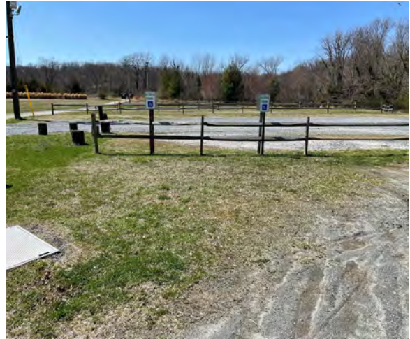
8.1.6. Accessible Parking spaces.
