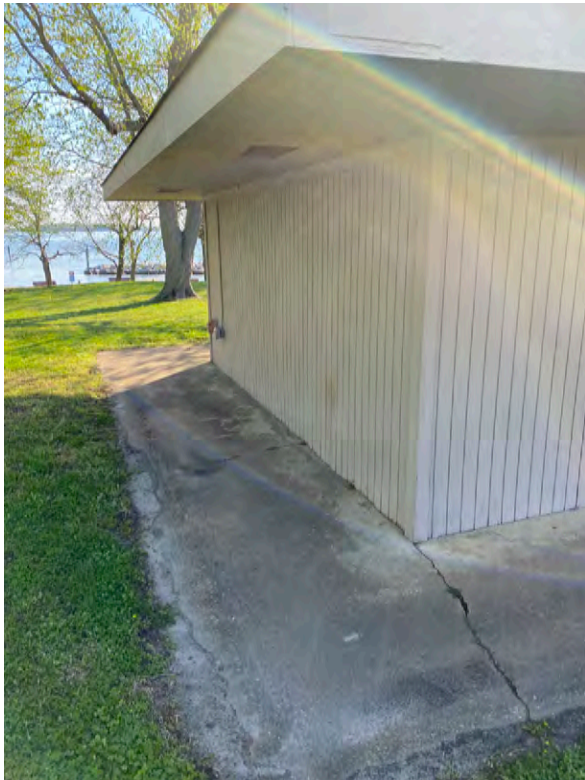
Concrete Apron and Siding
