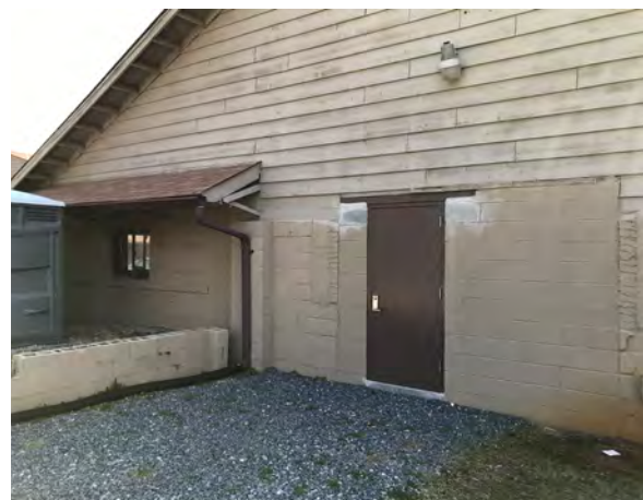
North Elevation Masonry Infill & Patching
