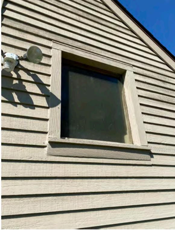
Wood-framed Window, Exterior View
