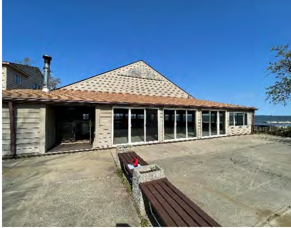
Exterior view of main entry
