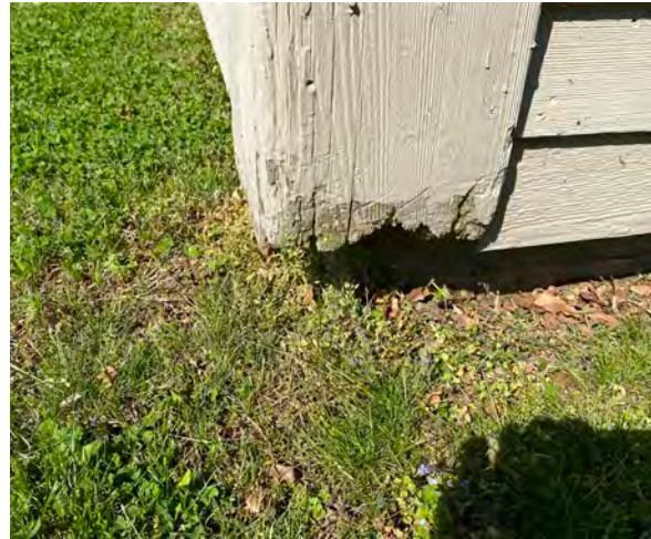
Exterior detail view
