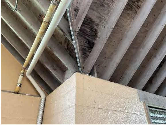
View of the valley conditions of Men's Room side.
