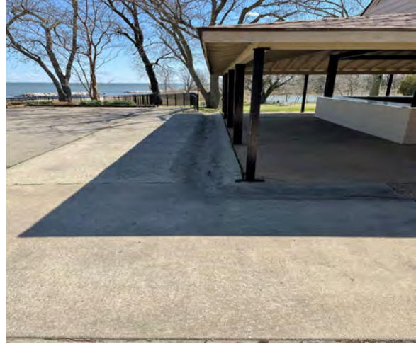
8.4.6 Drainage trough in sidewalk.
