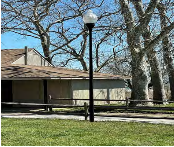
8.6.1 Existing site light poles.
