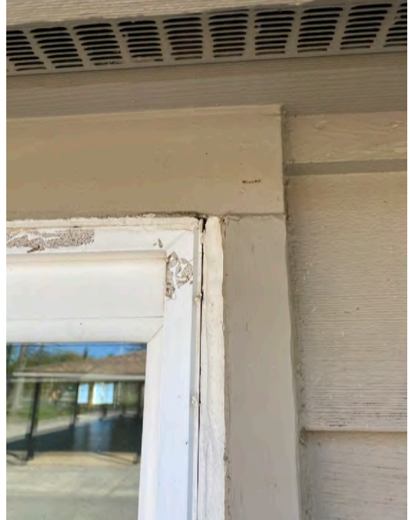
Deteriorated sealant
