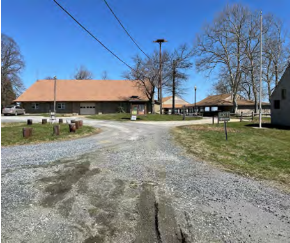
8.1.7 Gravel drive serving as the exit point from the parking area.
