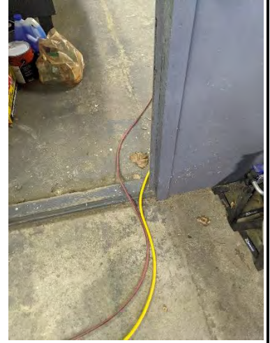
B: Unprotected Cord through door
