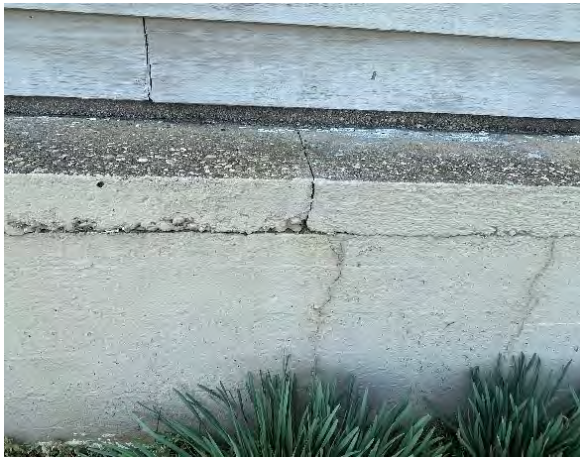
Exterior Foundation wall where slab projects
