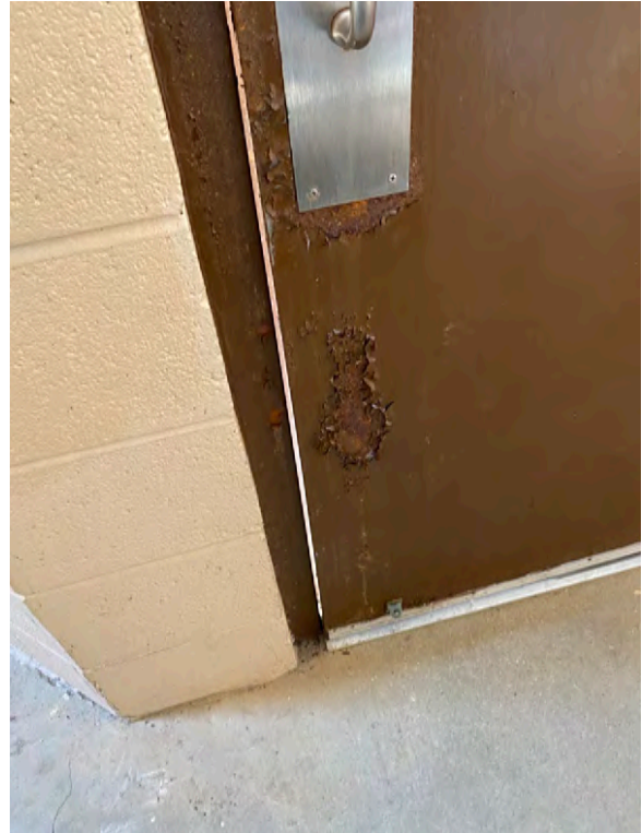
Door 702/A from interior
