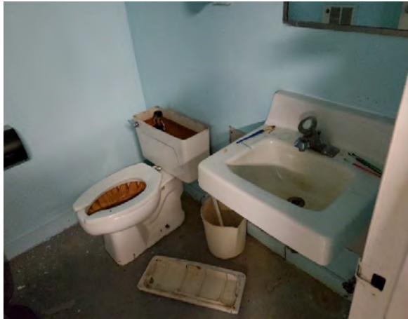
Bathroom 408 Lavatory and Water Closet
