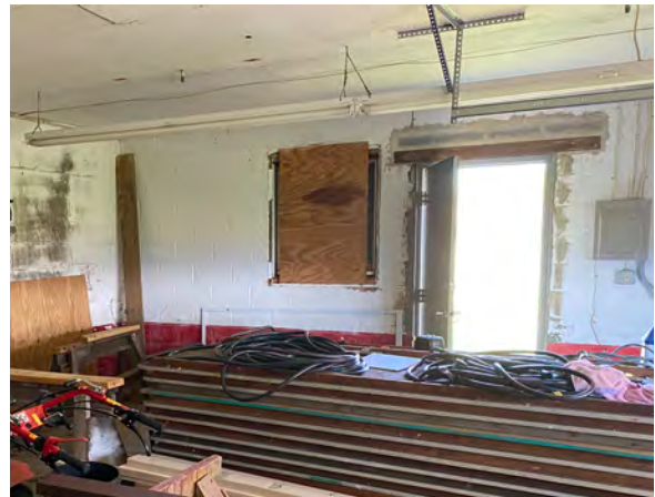
Interior view of entombed window opening
