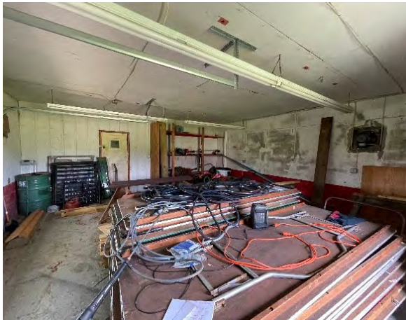
Interior view of work zone area.
