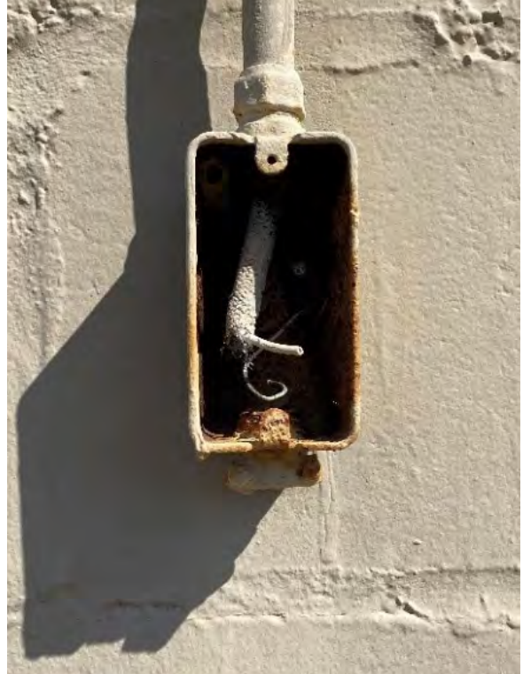
Exposed Wiring
