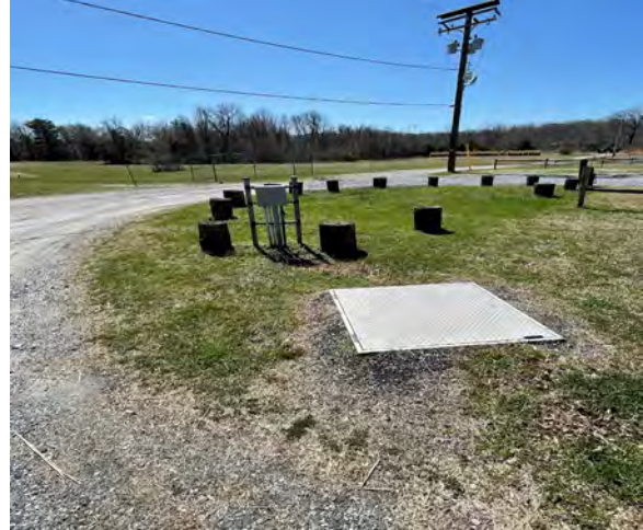
8.3.4 Existing septic pump.
