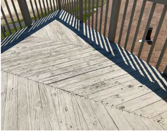
Balcony 215 - Deck boards
