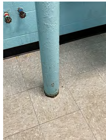
View of column base in bathroom
