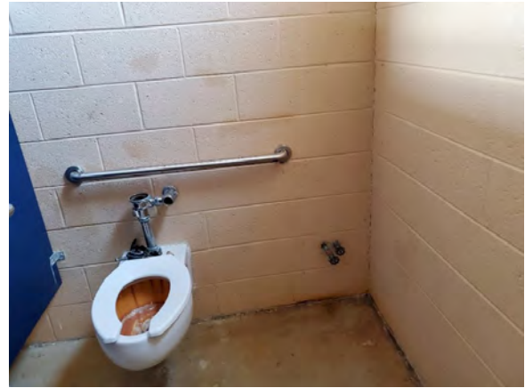
Men's Bathroom Water Closet
