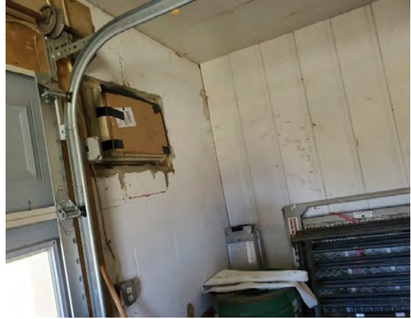
Through the Wall Unit Sleeve
