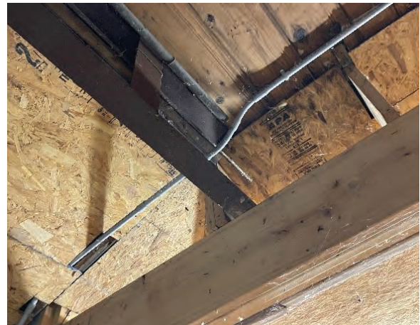
View of header with steel frame bearing.
