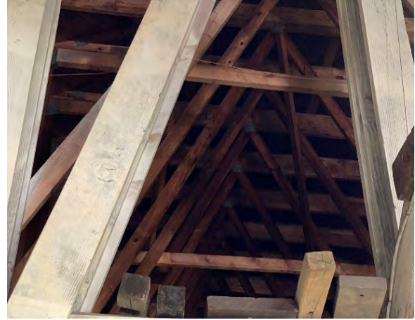
Limited view of clear span roof trusses beyond shop area.
