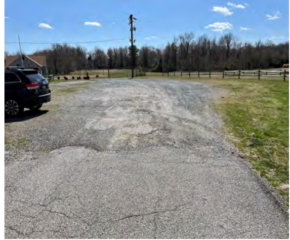
8.1.4. Transition from paved entrance drive to gravel parking area.
