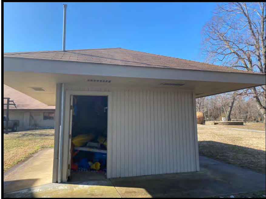
11. Storage Building 1 (dog house)
