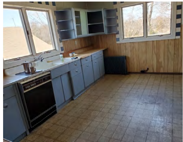
Second Floor Kitchen Sink
