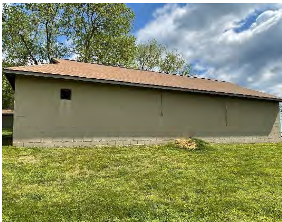
Exterior Elevation - South; note the mounded dirt.
