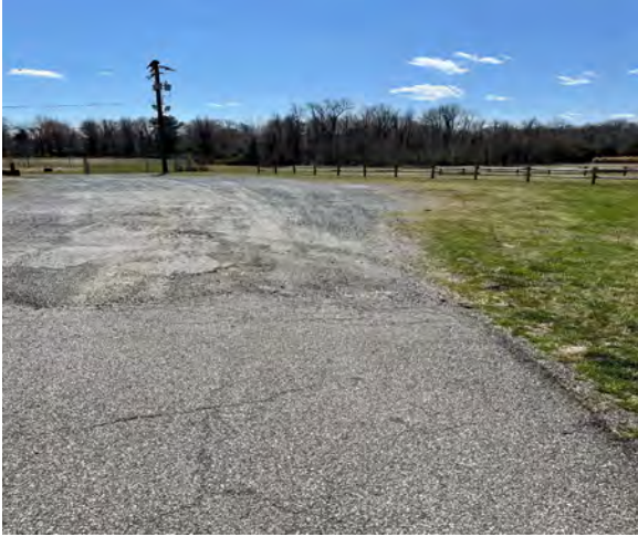
8.1.3 Transition from paved entrance drive to gravel parking area.
