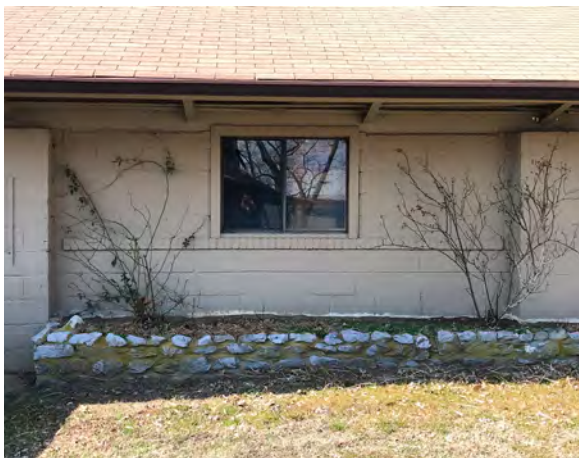
East Elevation Masonry Infill & Patching
