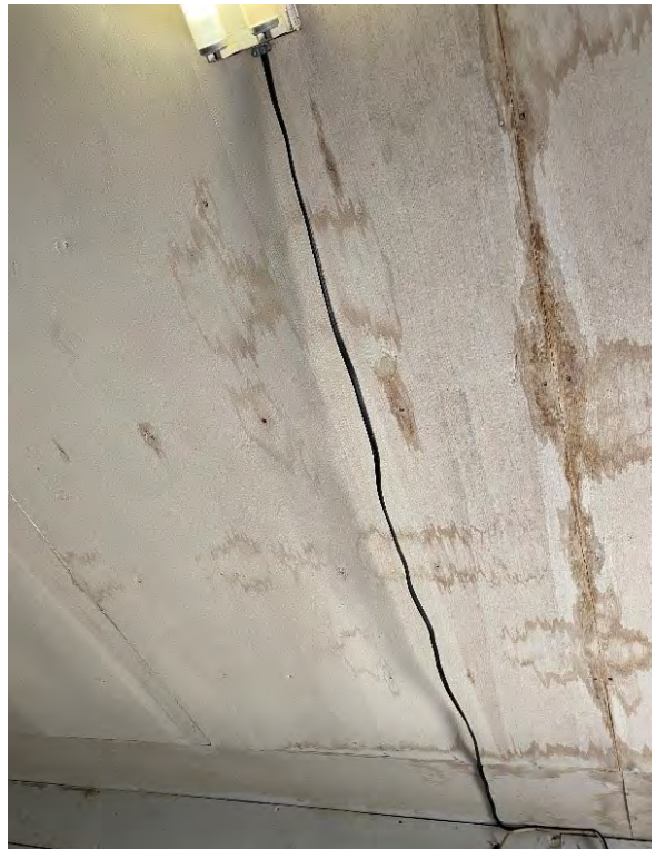
Typical Indoor Wiring
