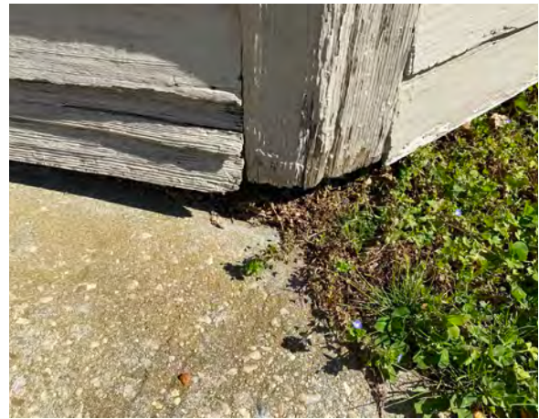
Exterior Wood Siding
