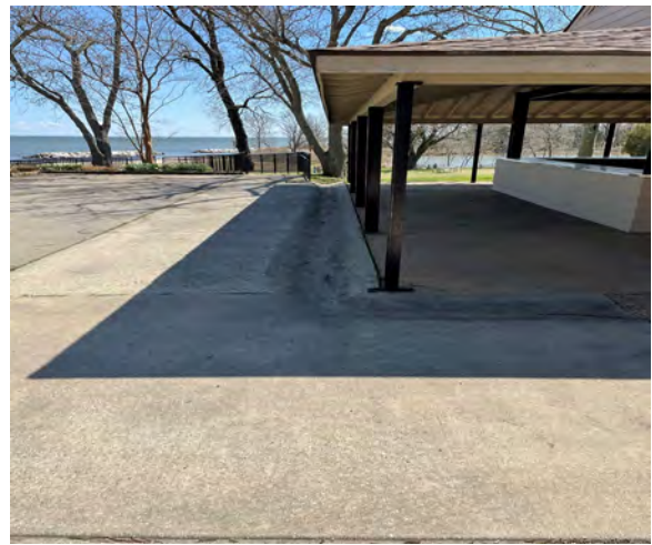
8.2.2 Example of concrete sidewalks around pavilion structures.
