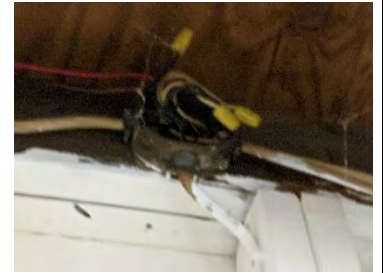
C: Missing junction box covers
