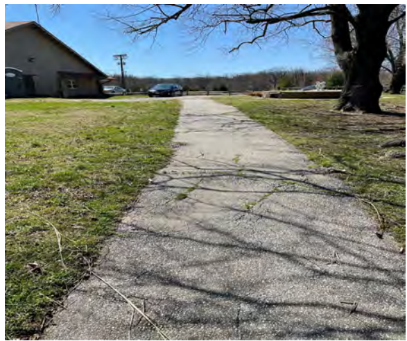
8.2.4 Existing asphalt pathway to Pavilion and Storage buildings (accessible route).
