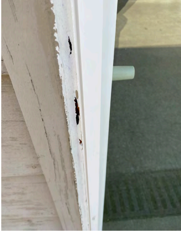
Deteriorated sealant
