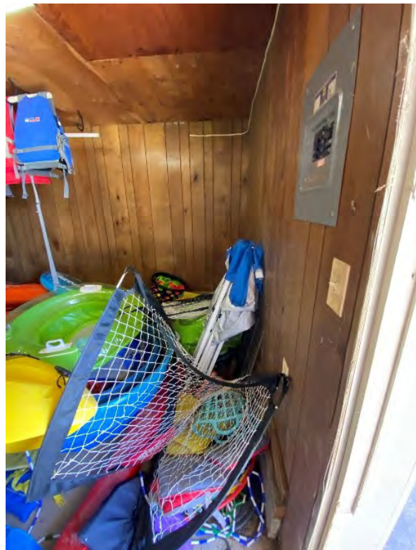
Load Center Working Clearance
