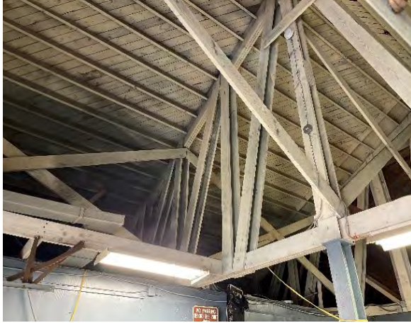
Interior view of timber trusses above shop area.
