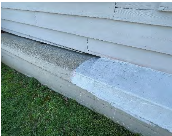
Exterior Foundation wall where concrete wash was installed.
