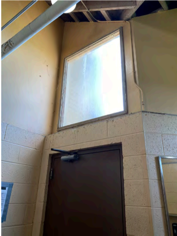
Wood-framed Window, Interior View
