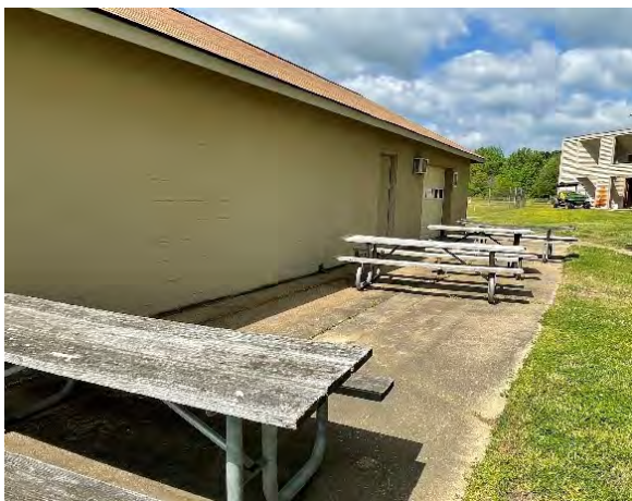
Exterior view of concrete apron slab.
