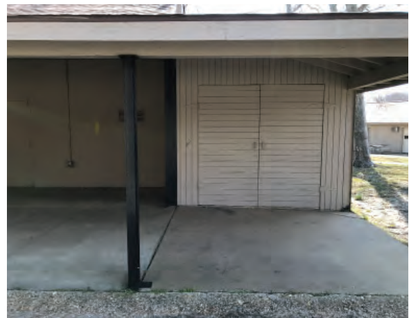
View of Concrete Floor and Steel Support
