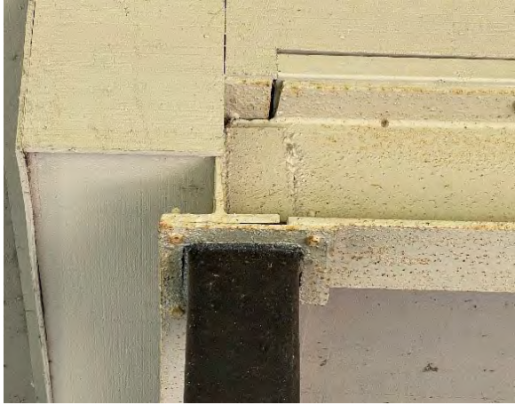
Exposed steel framing under second floor.
