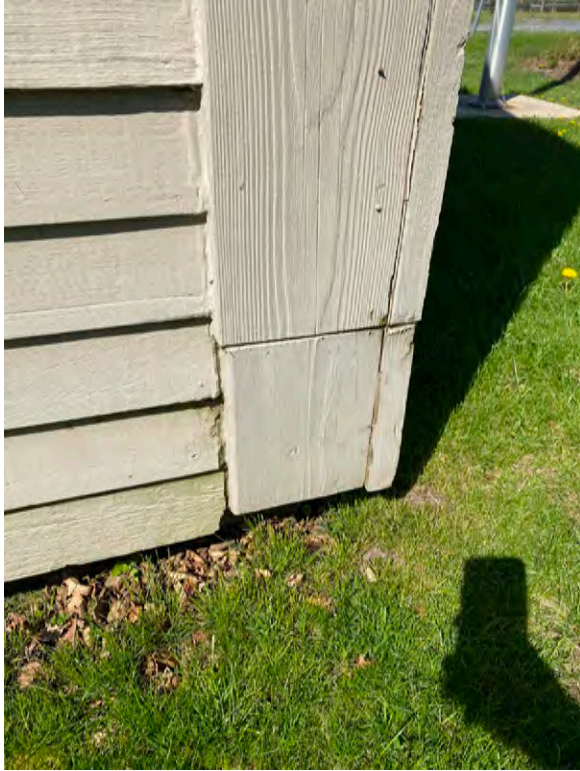
Wood Lap Siding - Prior Repair (Dutchman)
