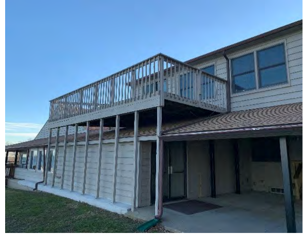
View of rear elevation facing the water.
