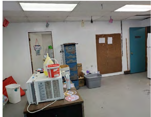
Window AC Unit in Office
