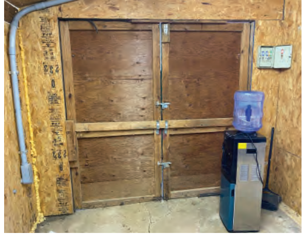
Wood Paneled Walls in Equipment Room
