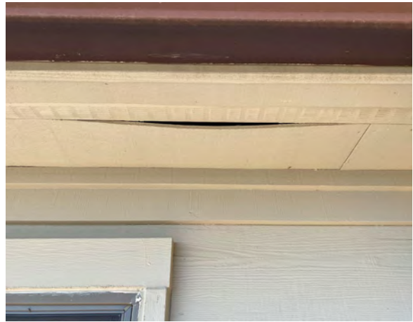
Soffit damage
