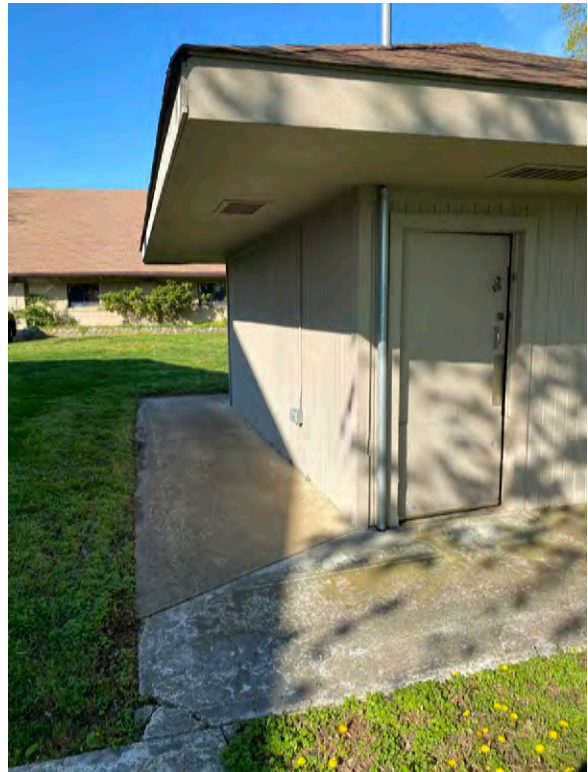
Door 501/A from exterior
