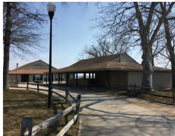
Exterior of Roof
