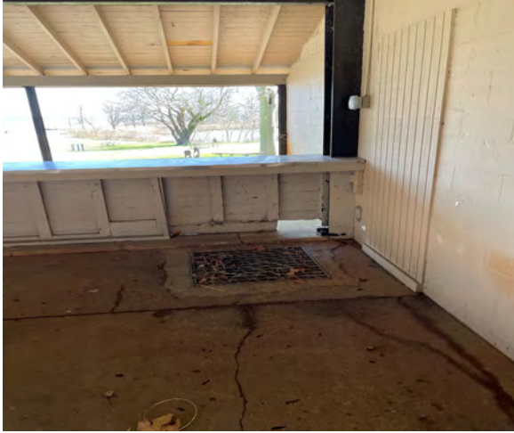
8.4.5 Storm inlet structure within the pavilion.
