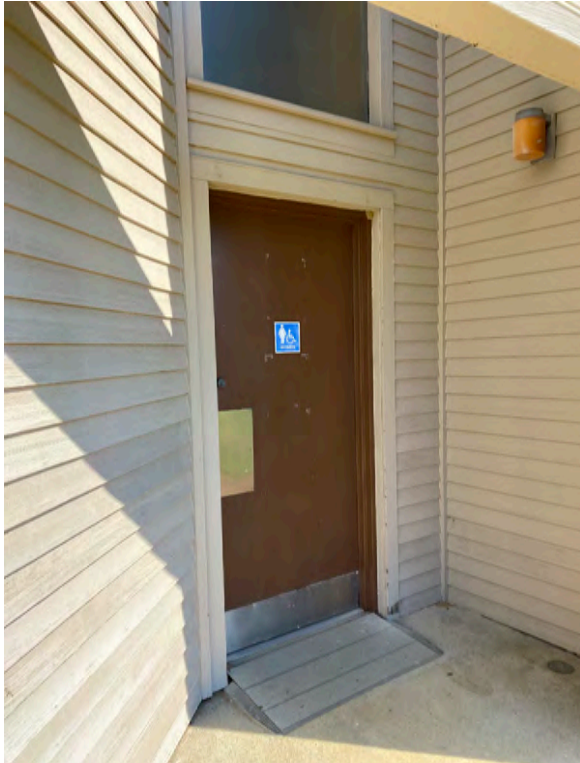
Door 701/A from exterior
