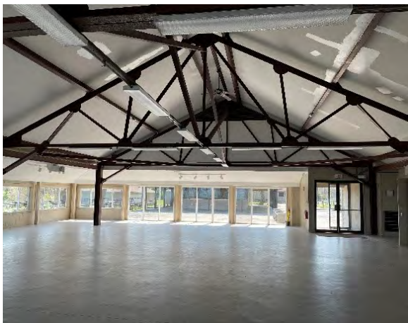
Typical interior view of main level
