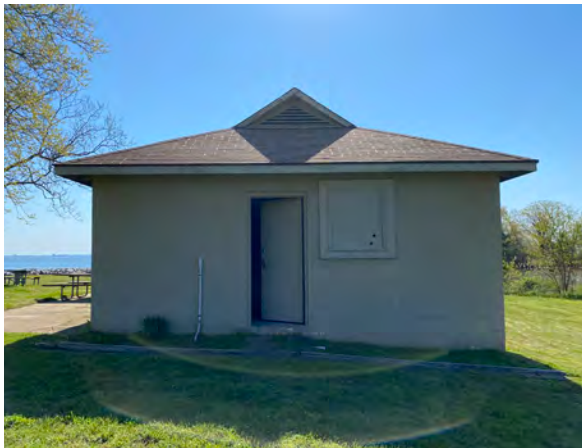
Exterior view of entombed window opening
