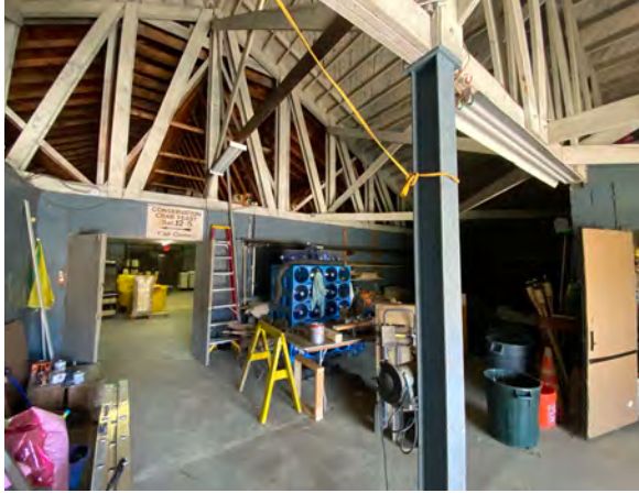
Room 402 - Open Ceiling
