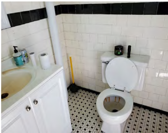
Second Floor Water Closet and Lavatory
