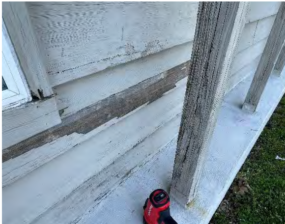
Exterior view of area below second level deck.
