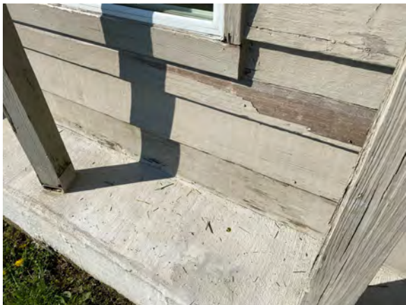
Deteriorated siding
