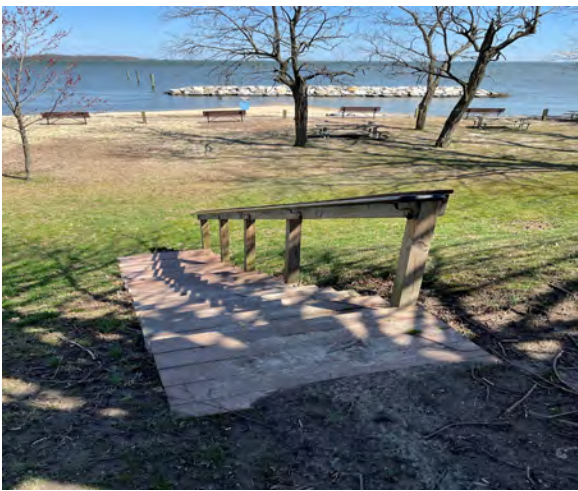
8.2.3 Existing stairs leading to playground.
