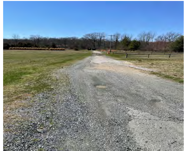
8.1.10 Existing gravel drive to service dumpsters.
