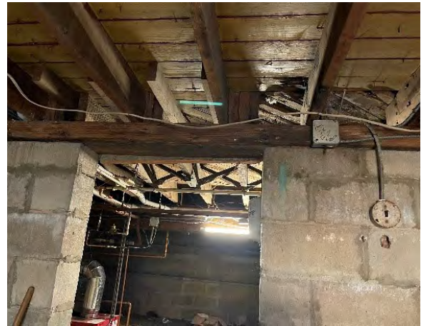
View of area where former water damage occurred.
