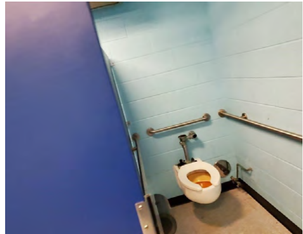
Men's Bathroom Water Closet
