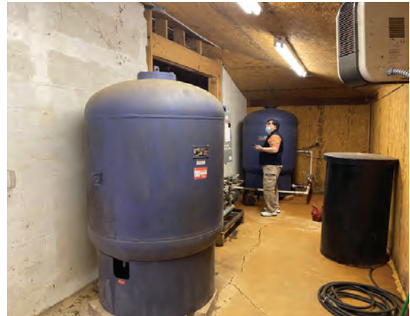
View of concrete floor
