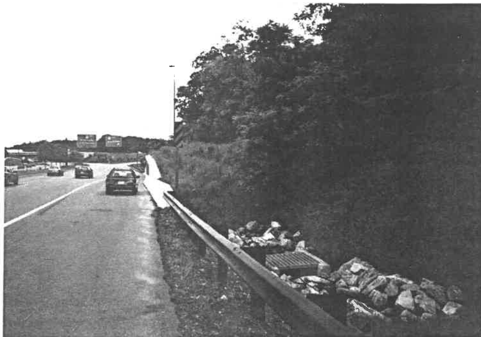
Rowe Boulevard Shoulder; Kirkley Road on Hill Behind Trees
