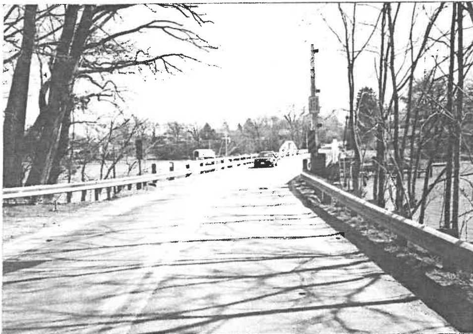
Ridgely Road Bridge Over Weems Creek
