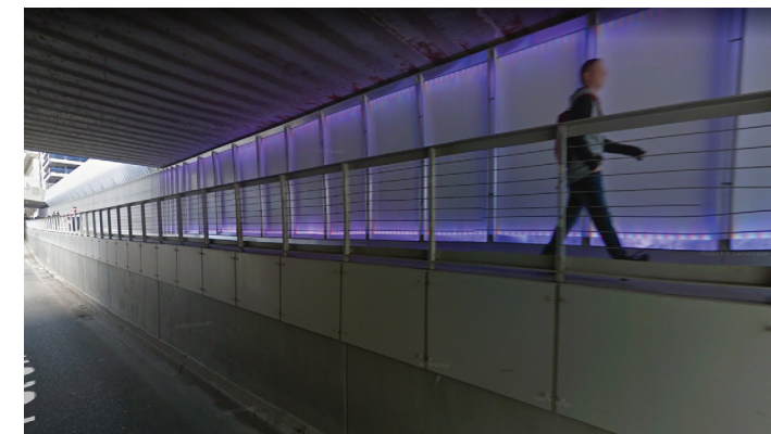
Artistic treatments enhance underpass environments for bicyclists and pedestrians. At top: "Phoenix Flowers" art installation and landscaped park beneath a freeway in Glasgow, UK. At bottom: colorful lighting along Calgary, Alberta's 4th Street underpass.
