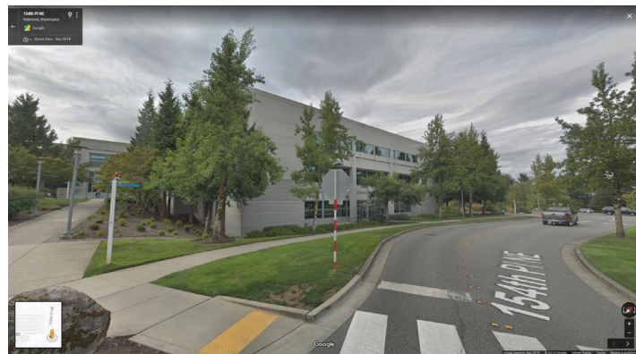
Office parks should offer attractive, well-landscaped settings, with bicycle, pedestrian and transit links to the rest of Parole, Annapolis and the region.
