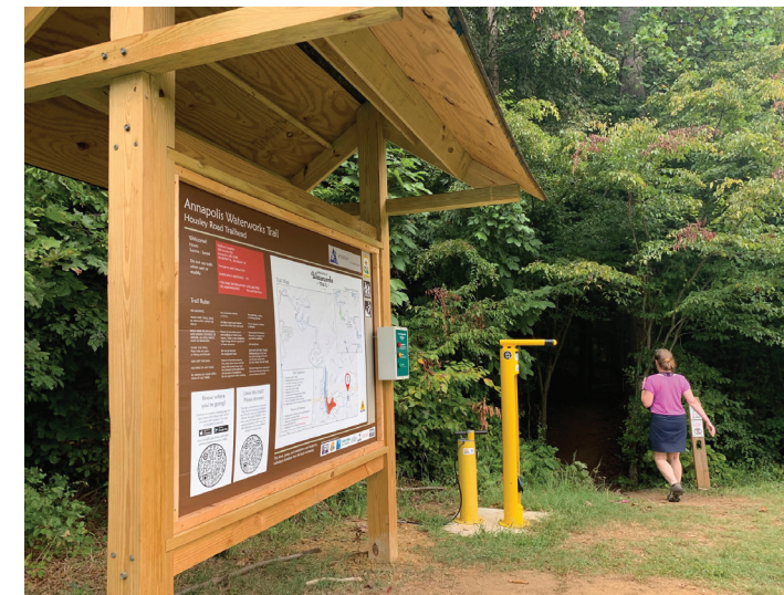
The City of Annapolis, in cooperation with private groups, recently constructed a trailhead to access the miles of hiking and biking trails and recreational areas of Waterworks Park, on the western edge of Parole Town Center.
