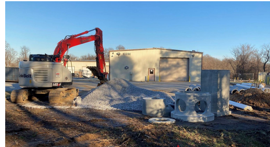
Millersville Landfill Warehouse Renovations (2022)
