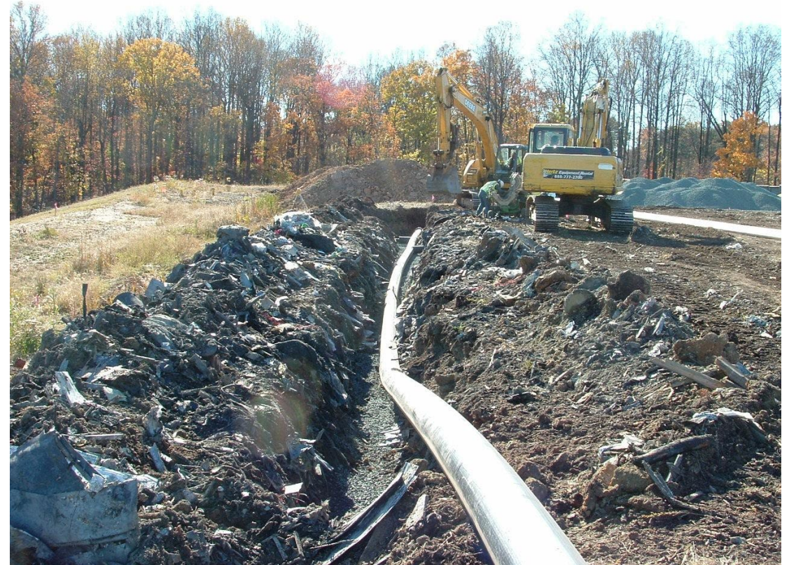
Temporary Gas Collection System Install Subcell 9.1
