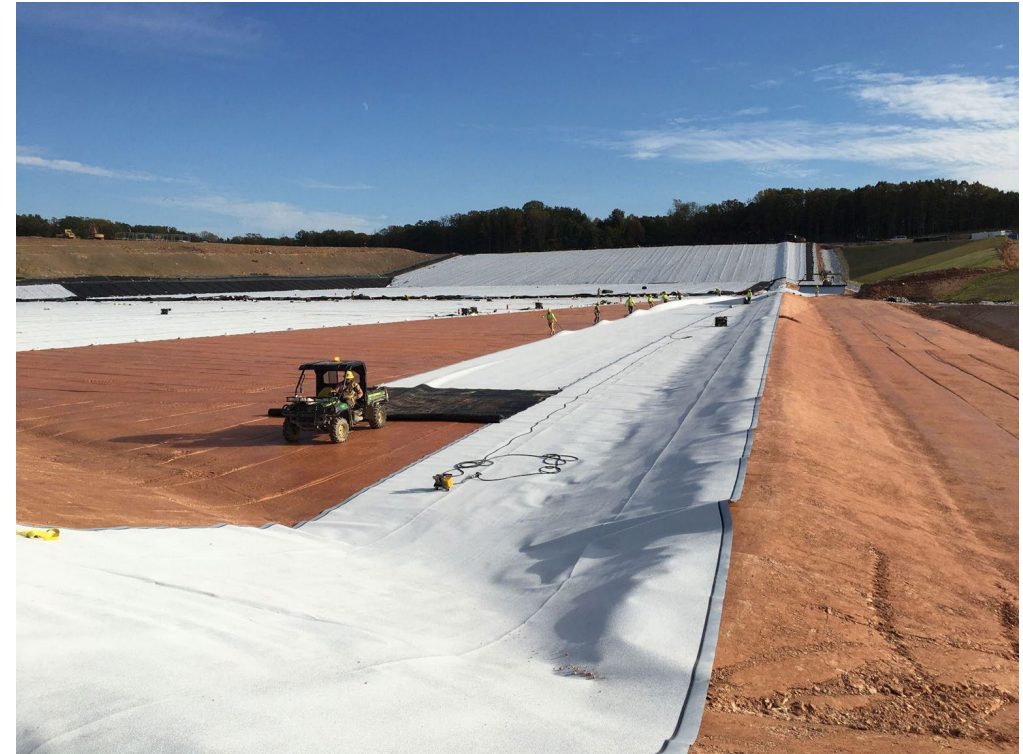
Geosynthetic Bottom Liner Deployment - Subcell 9.2
