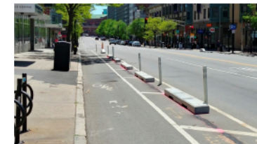
Figure 4: A separated bicycle lane located in Boston, MA. Source: Toole Design Group.
