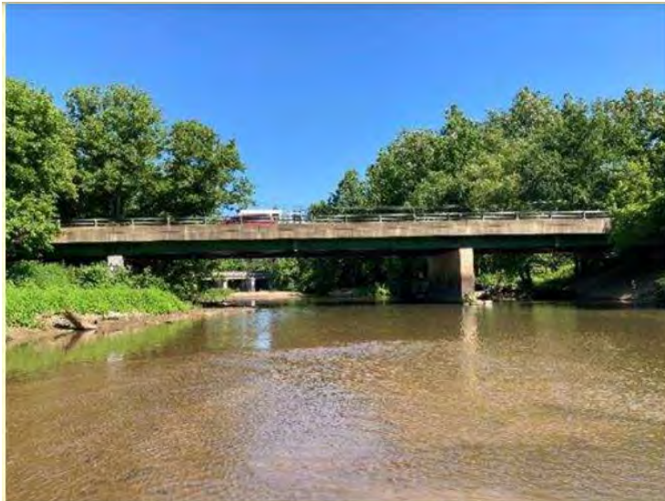
BRIDGE NO. AA4004001 PATUXENT ROAD OVER LITTLE PATUXENT RIVER
