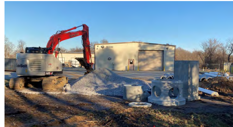
Millersville Landfill Warehouse Renovations (2022)
