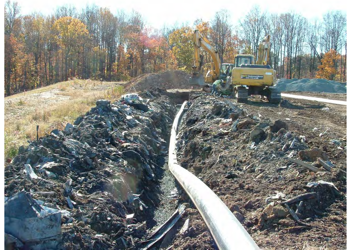
Temporary Gas Collection System Install Subcell 9.1
