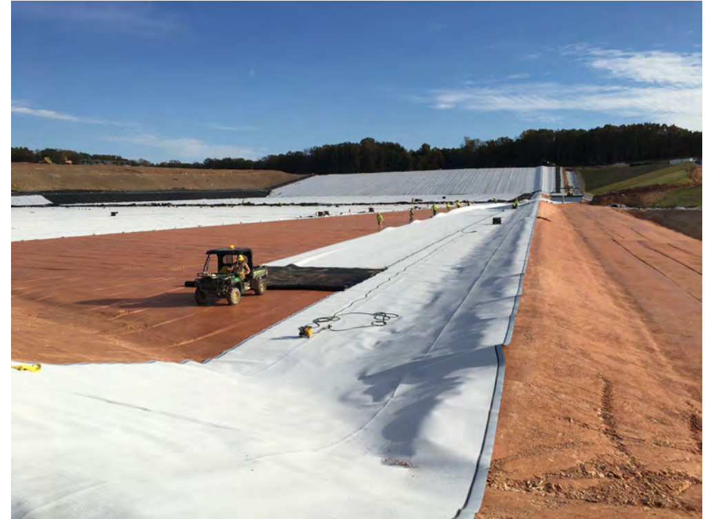
Geosynthetic Bottom Liner Deployment - Subcell 9.2
