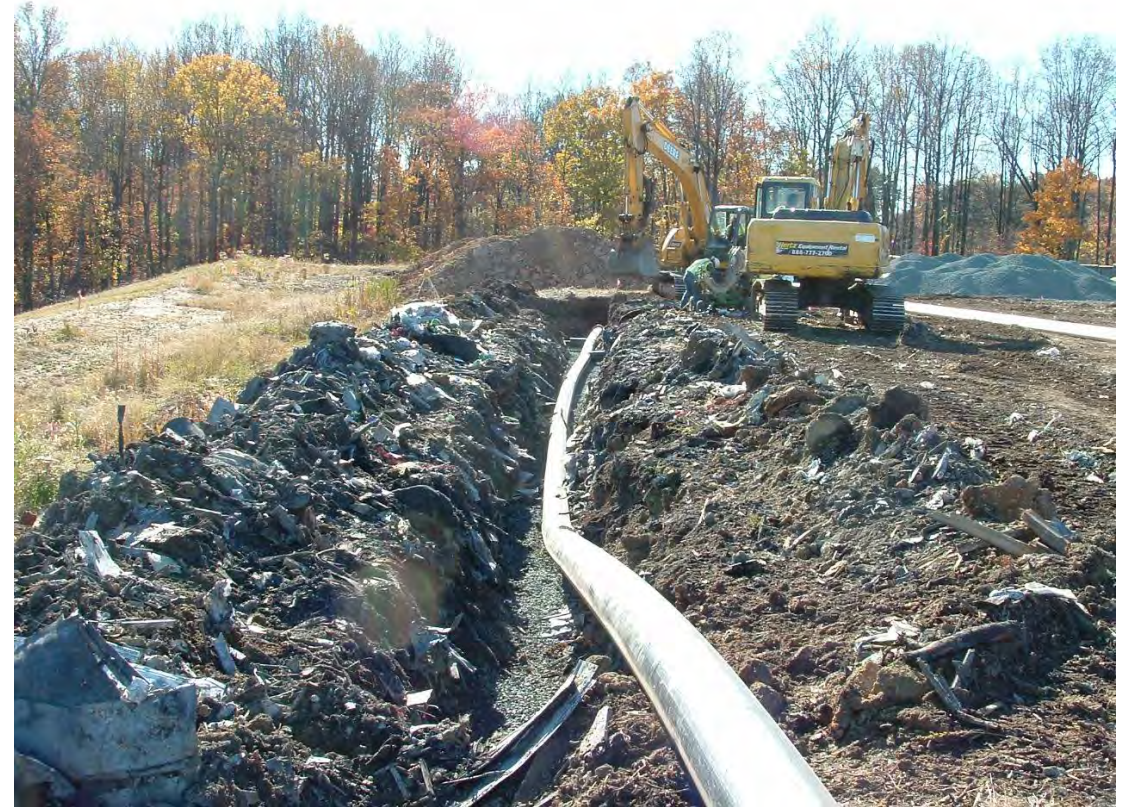
Temporary Gas Collection System Install Subcell 9.1
