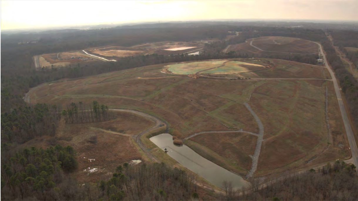
Cell 567 Closure Cap Repair (2020)
