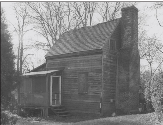
This mid-19th-century house is one of the few surviving examples of typical housing for enslaved workers, freedmen, and tenant farmers. Often just one room with a loft, for an entire family, these simple frame dwellings once dotted the landscape.
