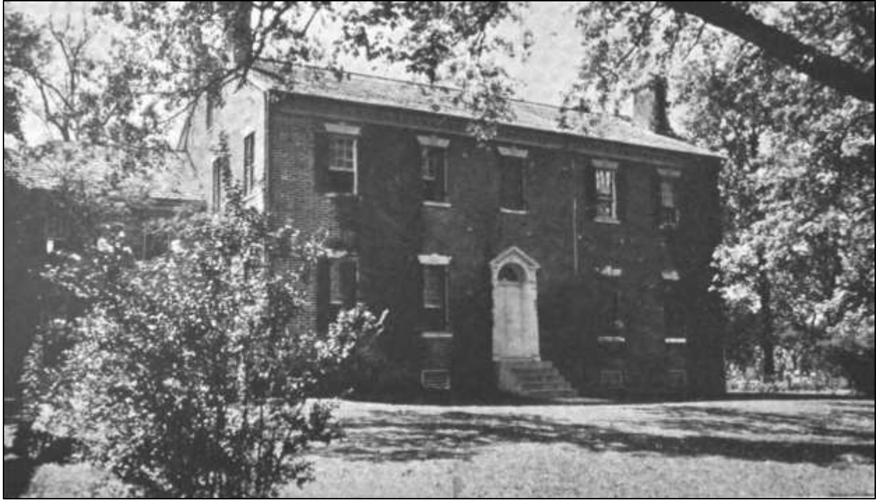
Figure 1 – Philip John Thomas had his house, Lothian, constructed in 1804 in the Georgian style as a two-story, side passage residence. The two bays on the right were added in the 1850s to create a symmetrical composition. (Katherine Scarborough, Homes of the Cavaliers , New York: Macmillan, 1930, after page 226)
