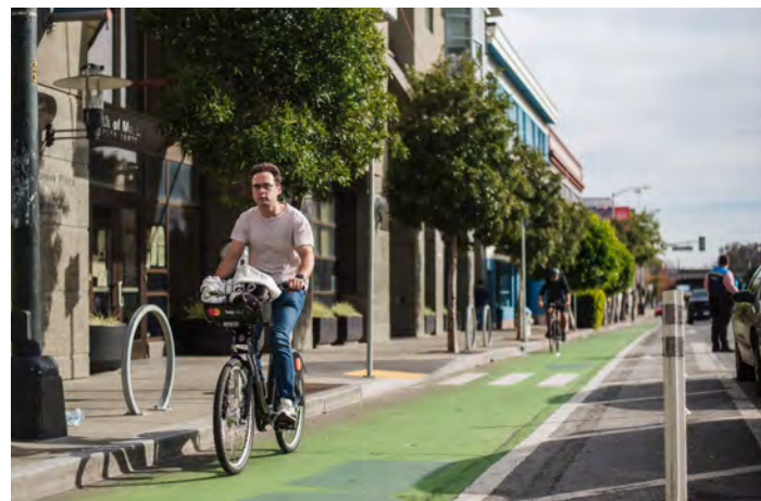
Figure 26: A separated bicycle lane. Taken by Toole Design staff.
