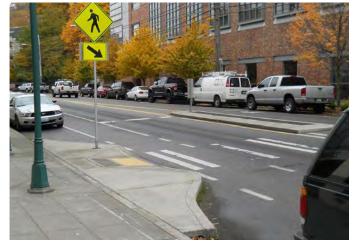
Figure 31: A bulb out is a feature of a high-visibility crosswalk. Picture taken by Toole Design Staff.
