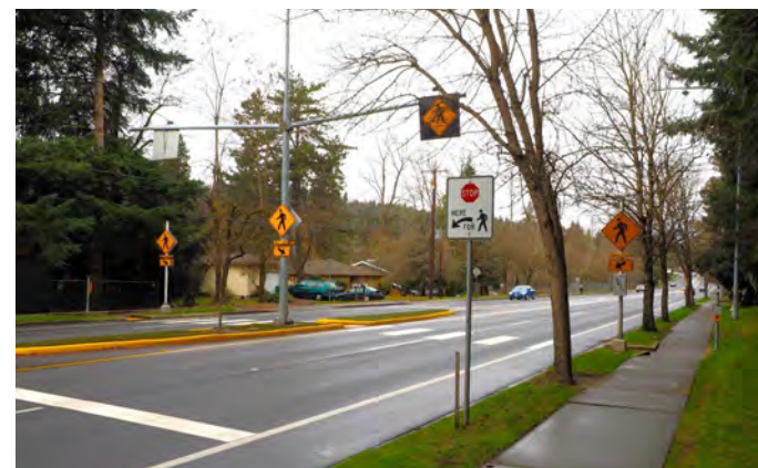
Figure 29: A Rectangular Rapid Flashing Beacon. Picture taken by Toole Design Staff.
