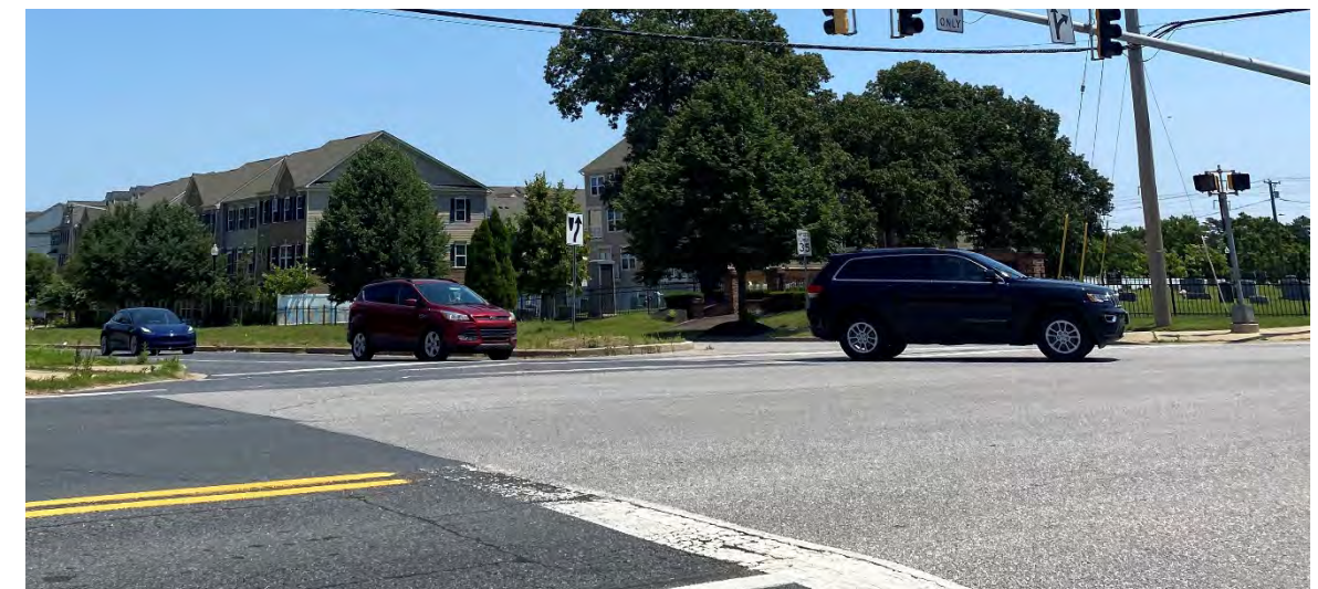
Figure 35: An intersection lacking crosswalks in Odenton. Taken by Toole Design Group.
