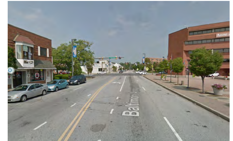
Figure 55: The existing cross section for MD 648, between MD 2 and MD 3. Photo from Google Maps.
