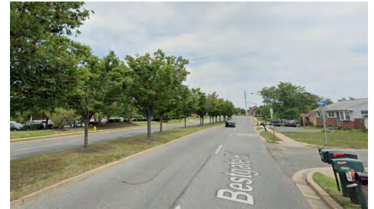
Figure 58: The existing cross section of Bestgate Road. Photo from Google Maps.
