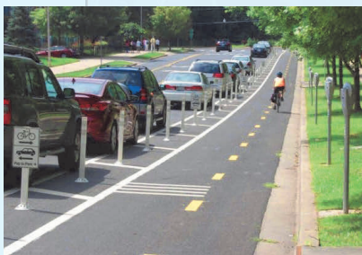
A Protected Bike Lane is a combination of horizontal separation (buffer distance) and vertical separation (e.g. flex posts, bollards, landscaping, curbs, etc.) to protect people bicycling from motor vehicle traffic. The combination of lateral buffer distance and vertical separation elements (such as flexible delineators, curbs or height differences, or vehicle parking) can ameliorate most of the stressors of on-street bicycling while taking advantage of the already paved surface.
