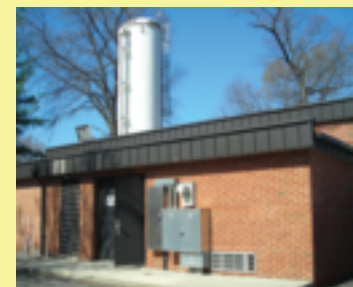
Glendale Water Treatment Plant
