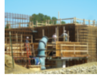
Construction at the Crofton Meadows WTP
