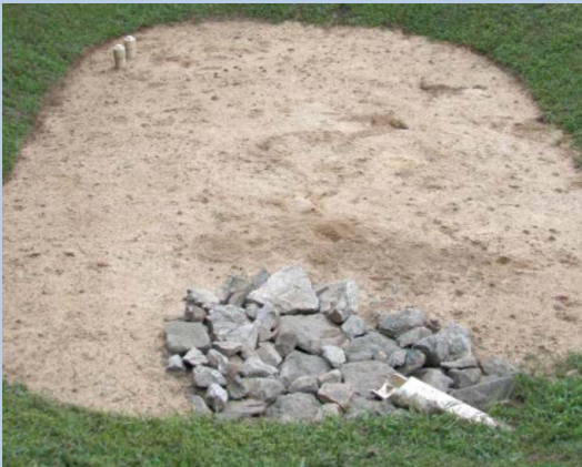
Typical surface sand filter
