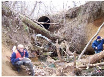
Looking up stream from original outfall location.
