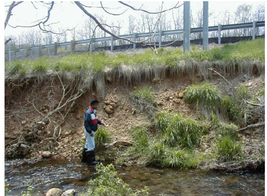
Before Restoration – Rosgen G Channel
