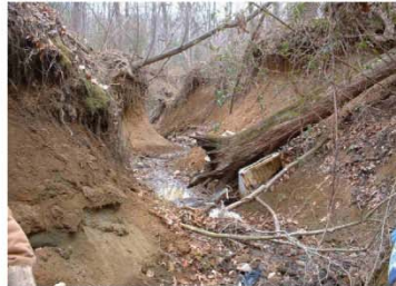
Looking down stream from original outfall location.
