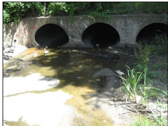
Photo 4 – Three Culverts Conveying Flow under McKinsey Road
