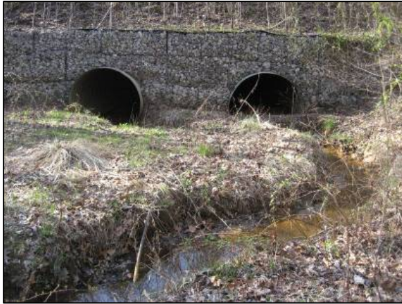
Photo 6 – Twin Culverts Conveying Flow From Under West Campus Drive
