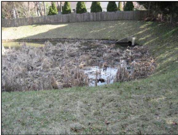
Photo 1 - Existing Infiltration Basin
