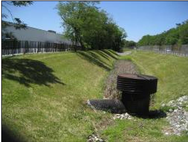
Photo 3 – Ditch and riser looking up gradient
