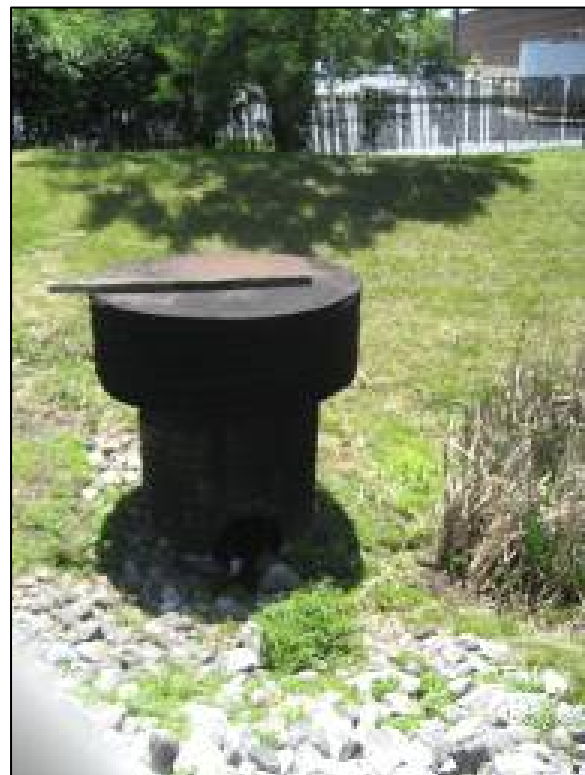
Photo 2 –Riser with bypass
