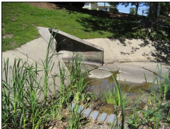
Photo 3 – Storm Outfall to Ditch near the End of the Proposed Retrofit
