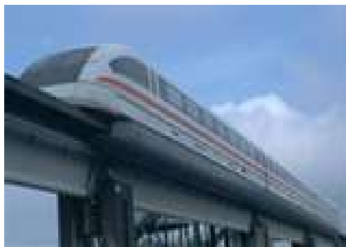
MagLev Train on Structure
