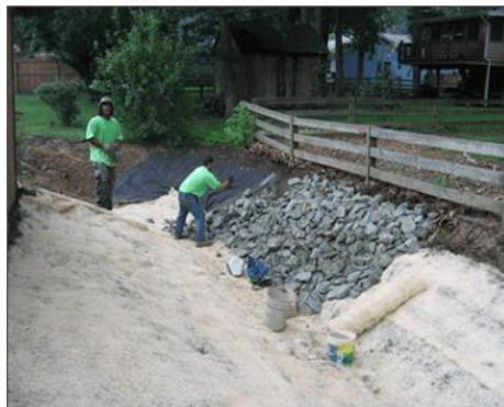
Figure 6.3-21 Rip-Rap Placed by Hand to Reduce Erosion (Source: Anne Arundel County website)
