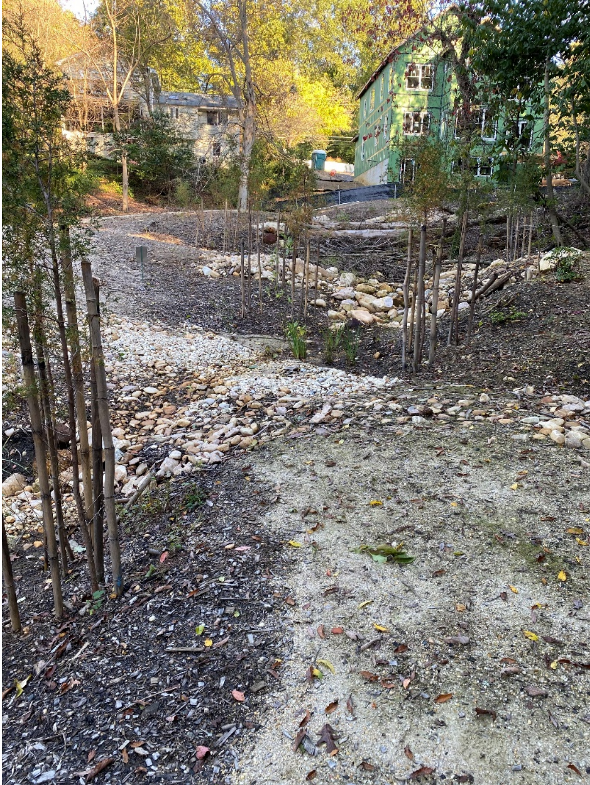
Figure B-7: Riffle weir sequence at Winchester SPSC (Anne Arundel County)
