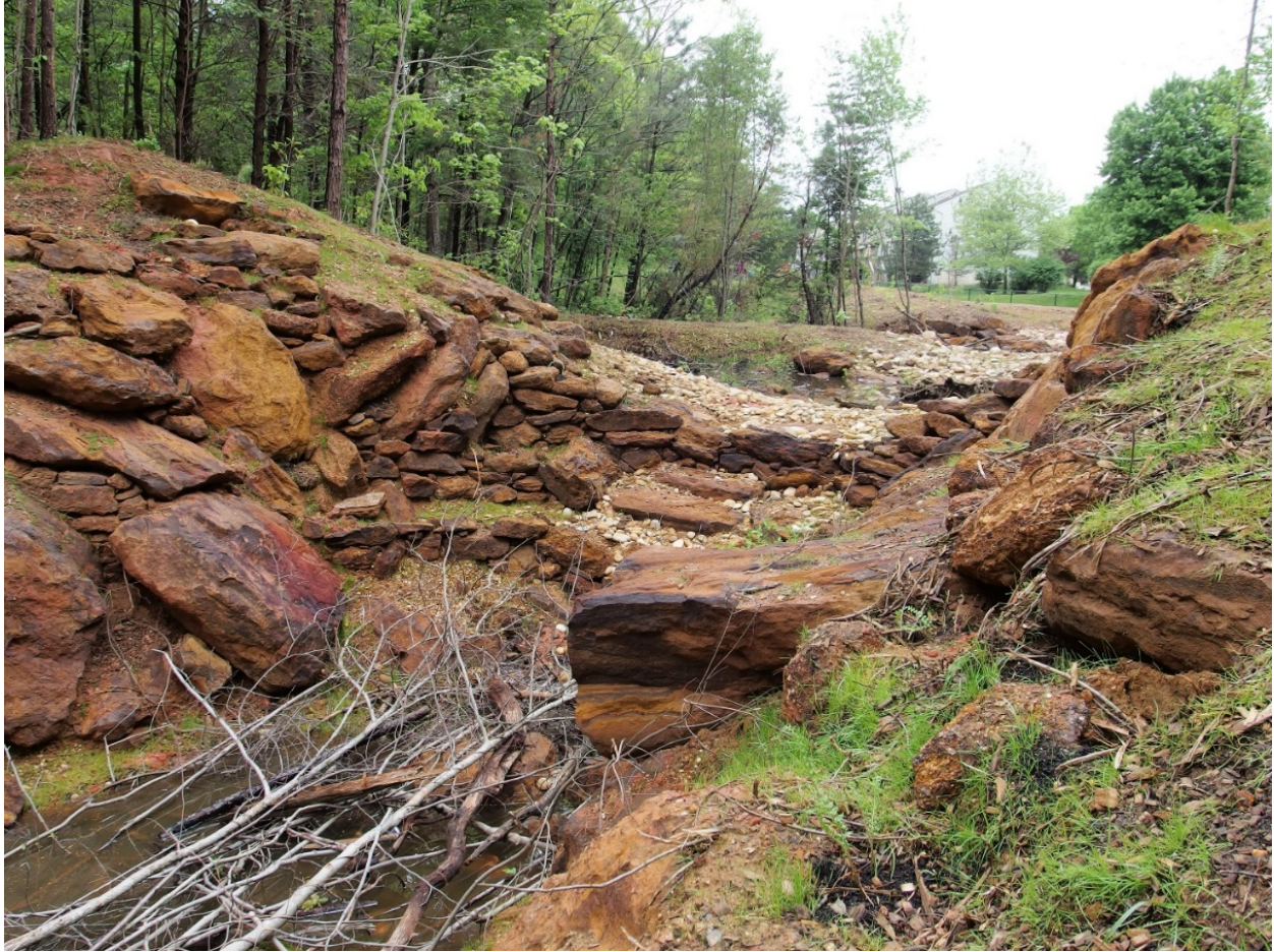
Figure 16: Hospital Drive SPSC, novel cascade weir design to navigate breach in former dam (Anne Arundel County)
