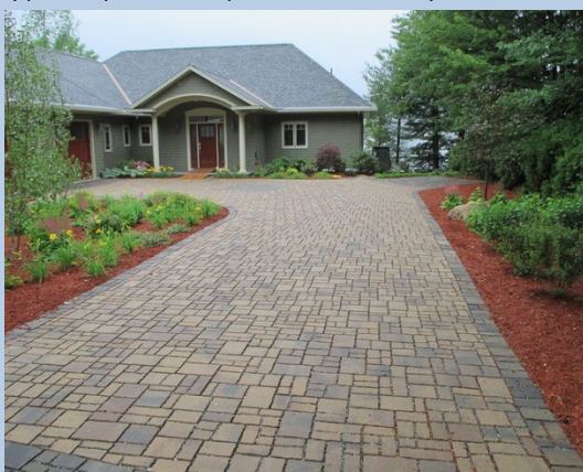
Typical pervious paver driveway
