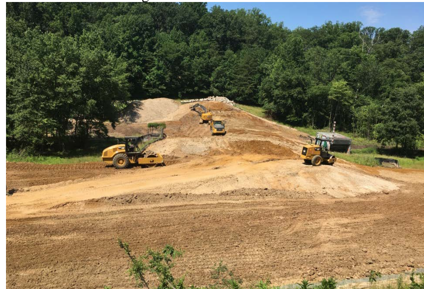
Photo 4 – Dam excavation and fill placement
