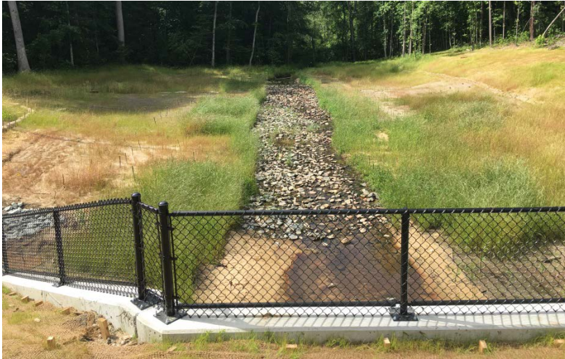
Photo 1 – View upstream from W Benfield Road and new box culvert
