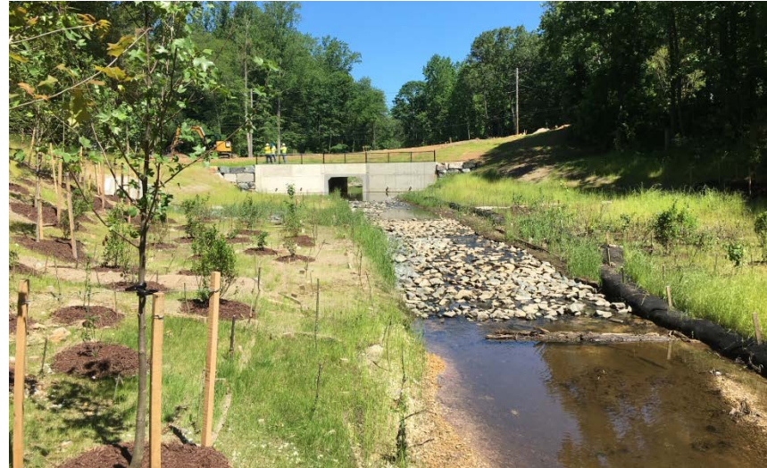
Photo 2 – Plantings downstream from the new culvert
