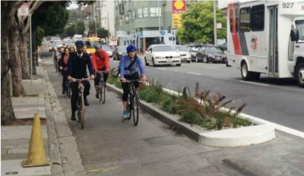
**Separated Bike Lanes:** Separated bike lanes are similar to buffered bike lanes except that they are characterized by some sort of vertical barrier, such as bollards, planters, or even parked cars.
