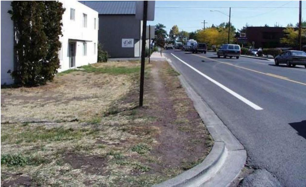
**Buffered Sidewalk should replace worn paths that show desired walking locations.**
