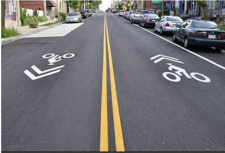
**Shared Lane Markings, or “Sharrows,”** are used to indicate a shared lane environment for bicycles and automobiles. These should most often be used on low speed roads, where space constraints may be present.
