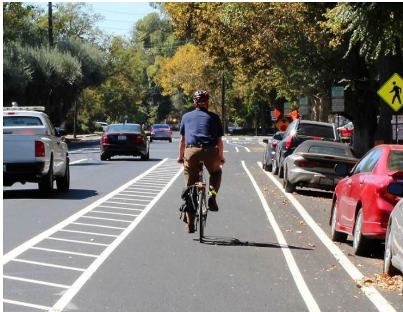
**Buffered Bike Lanes:** Conventional bicycle lanes paired with a painted designated buffer, characterized by two vertical lines and hatching. This image shows a buffer to both the automobile travel lanes and the parked cars.
