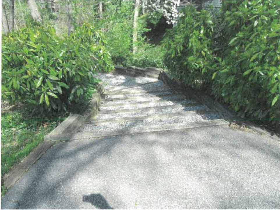
Figure 7: Ex. Stairs to Basement Entry
