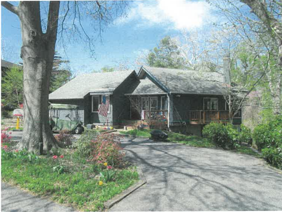
Figure 1: Front of House Looking SE
