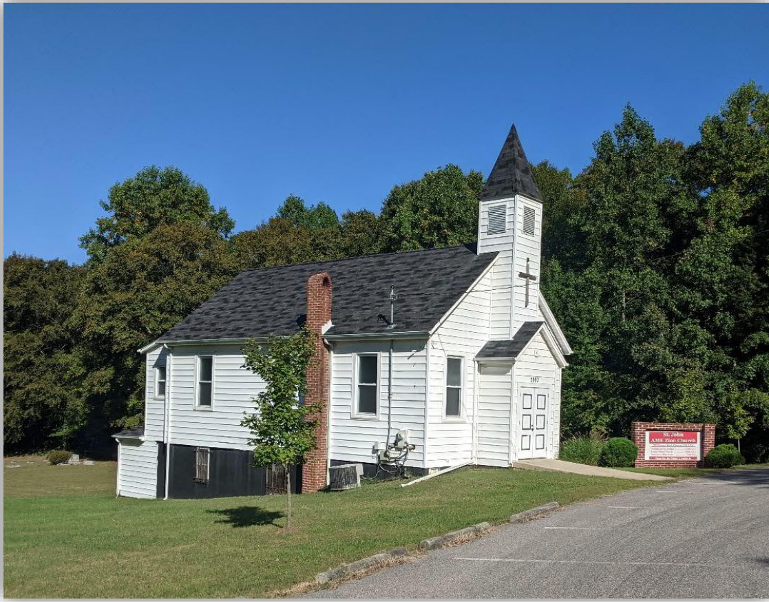
Figure 2-8: St. John A.M.E. Zion Church, located at Western Terminus of Conway Road
