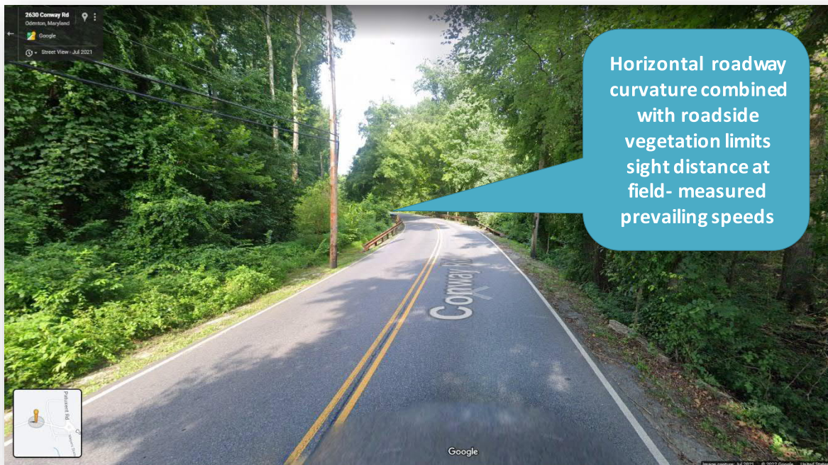
Figure 5: Example of Limited Sight Distance on Conway Road west of Patuxent Road
