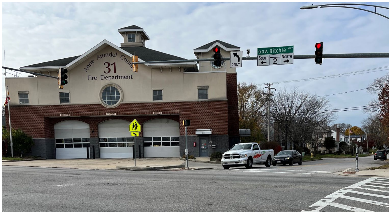
Figure 1 Anne Arundel County Fire Station # 31 at 11th Street and Ritchie Highway in Brooklyn Park, MD
